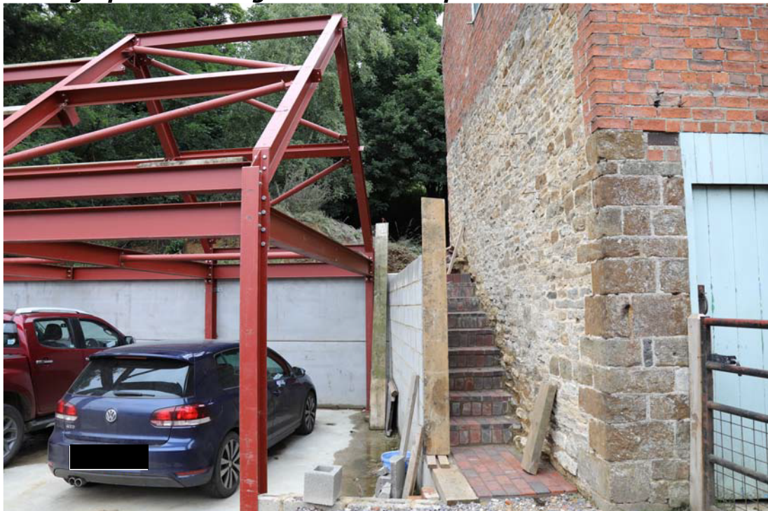
Photograph 2: Existing listed brick steps
