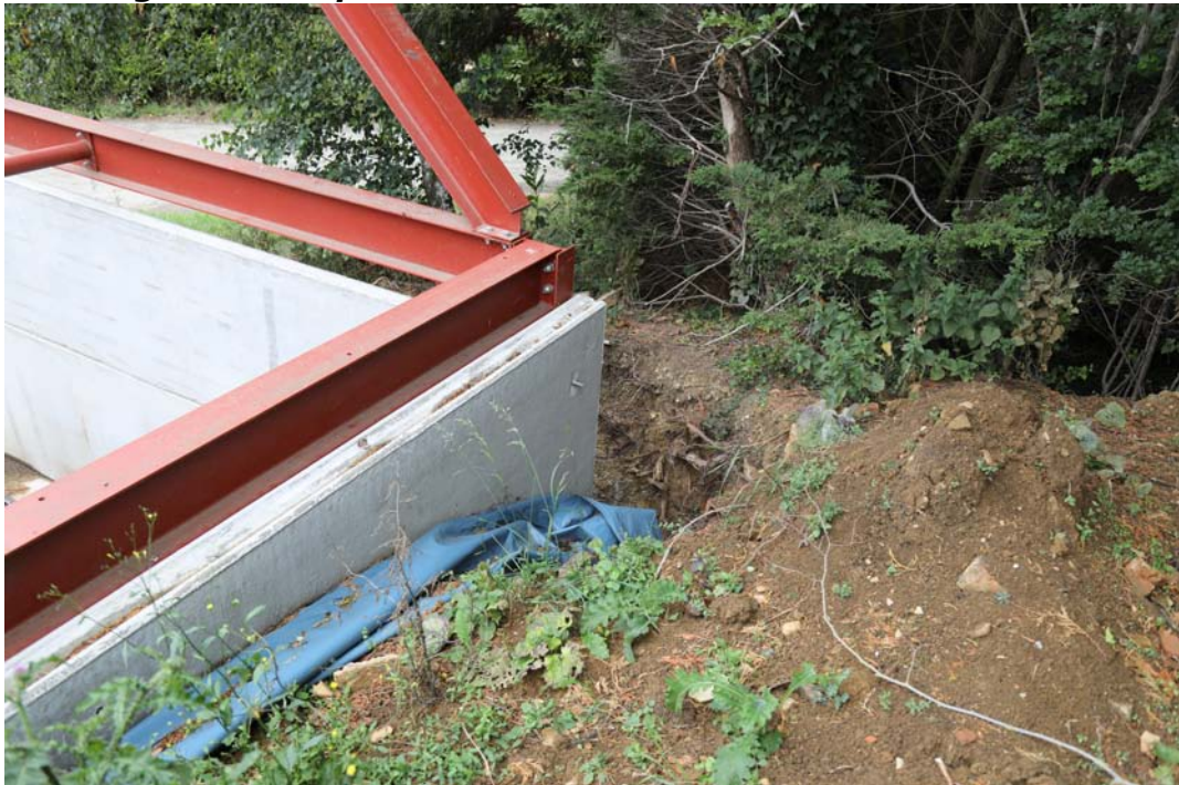
Photograph 4: North-west corner from atop the earth bank showing concrete planks
