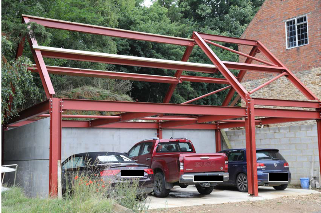
Photograph 1: The steel frame of the carport and workshop
