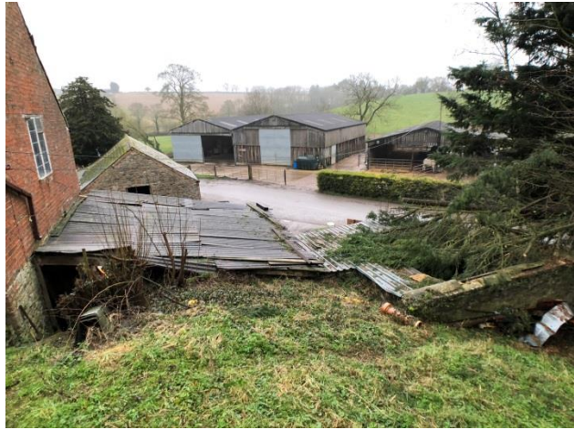
Photo 3: The rooves of the lean to and garage
