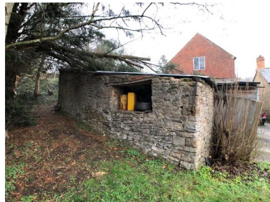
Photo 2: West elevation of the stone garage
