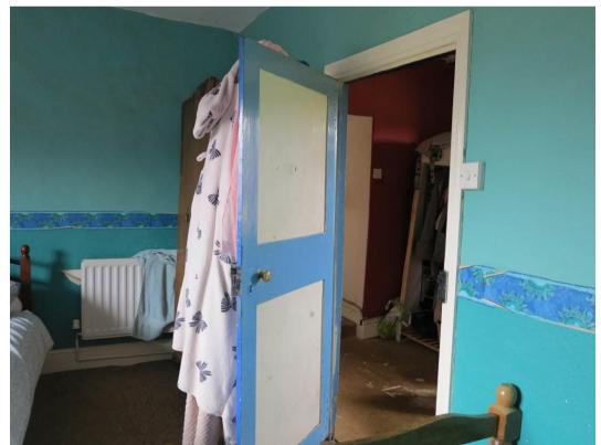
Plate 13. Inserted partition wall between lobby to bathroom and bedroom at east end of house; the 18<sup>th</sup>-century two-panel door must have been reused
