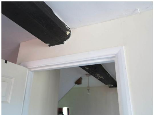
Plate 7. Note the way the ceiling beam runs through the inserted partition wall into the landing
