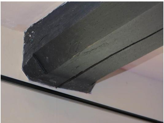
Plate 9. The stop end of the chamfered beam in the bedroom
