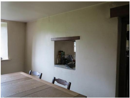
Plate 35. Former window in east wall of room below former granary
