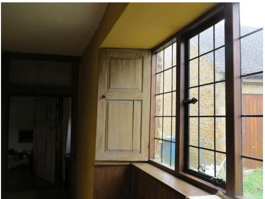
Plate 39. Internal window shutter in south wall of house
