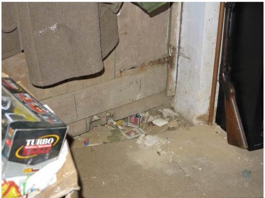
Plate 51. Strap hinges on reverse of plank door
