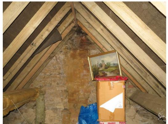
Plate 49. 20<sup>th</sup>-century roof structure of 19<sup>th</sup>-century single-storey addition
