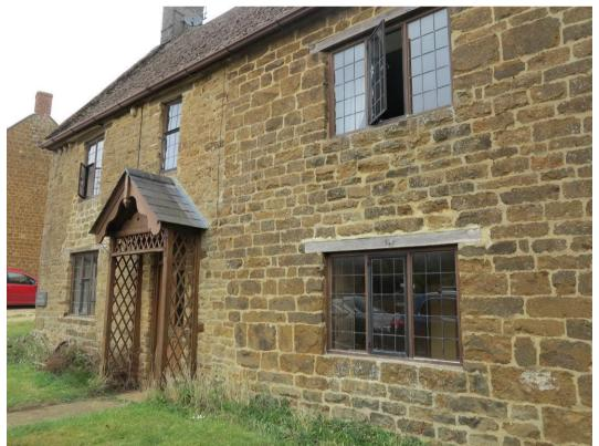
Plate 4. Burdrop Farmhouse, construction joint on south elevation
