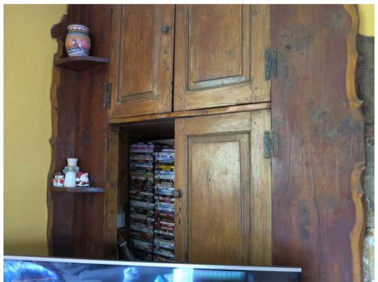
Plate 27. The alcove to the left of the inglenook fireplace, now infilled with a cupboard reusing 18<sup>th</sup>-century panelling, may be the location of an original staircase
