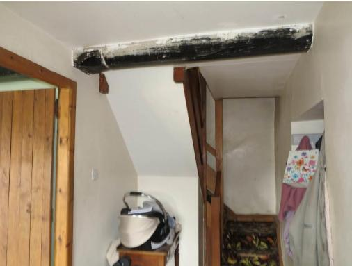
Plate 14. The wall separating the room at the west end of the house on the ground floor must be on a slightly different line from the original as the beam from this room carries through the wall to the present hallway
