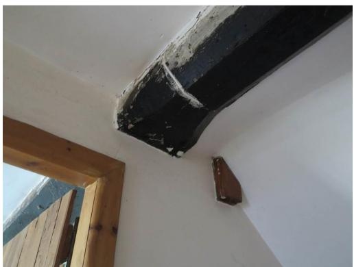
Plate 15. The wall separating the room at the west end of the house on the groundfloor must be on a slightly different line from the original as the beam from this room carries through the wall to the present hallway (detail)
