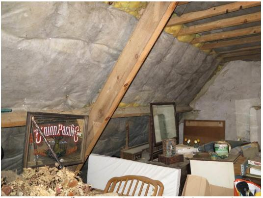
Plate 47. 20th-century roof structure in attic (east room)
