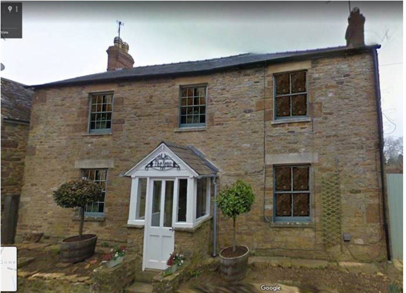
Changed the two windows on the right to show the proportions also work with 2 over 2.
