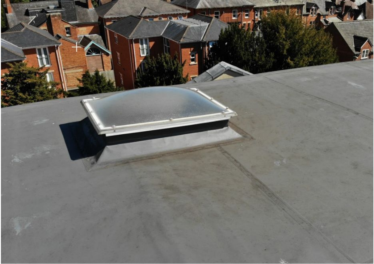
Current Roof Light
