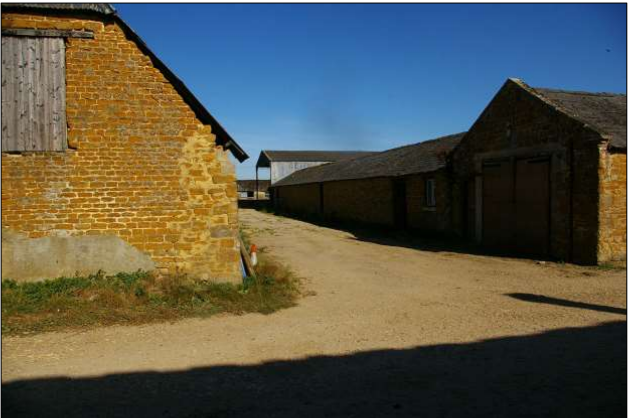
VIEW PAST THE THRESHING BARN TO THE U-SHAPED RANGES; VIEWED FROM THE WEST-NORTH-WEST.
