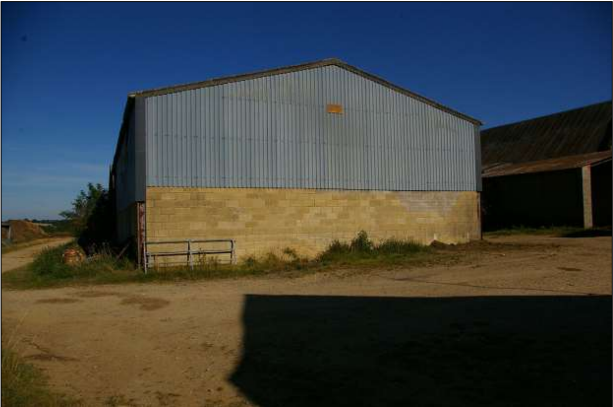
VIEW OF ONE OF THE LARGE MODERN AGRICULTURAL SHEDS, THAT FRAMES THE HISTORIC BARN ON THEIR NORTHERN SIDE; VIEWED FROM THE WEST-NORTH-WEST.
