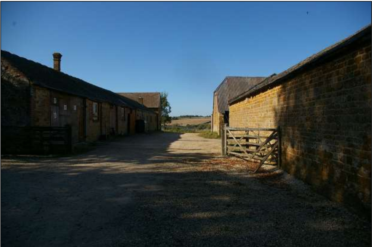
THE LATER RANGE OF BARNs AND WORKSHOPS TO THE WEST OF THE FARMYARD, WITH BRICK DETAILING, LIKELY MUCH LATER 19 TH CENTURY; VIEWED FROM THE SOUTH.
