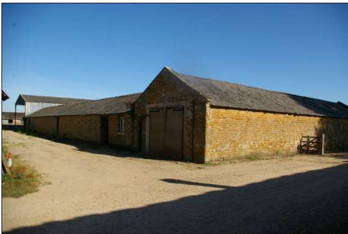
FIGURE 30: VIEW OF THE U-SHAPED FRONT RANGE OF BARNs AT HILL FARM THAT FLANK THE DRIVEWAY AND THE FARMHOUSE TO THE EAST; VIEWED FROM THE NORTH-WEST.
