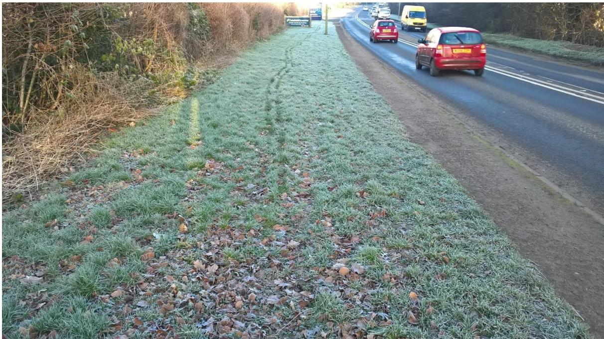
The highway boundary along this stretch is in the grass close to the back of the footway, so the area occupied by the layby and footway/cycletrack will need to be dedicated as highway. The works will be agreed and carried out under a S278 agreement. It is not proposed to have a southbound stop due to the lack of space on the other side of the A4260, but one may be introduced nearby, possibly in the existing layby, at a later date when the Longford Park Phase 2 is delivered.
