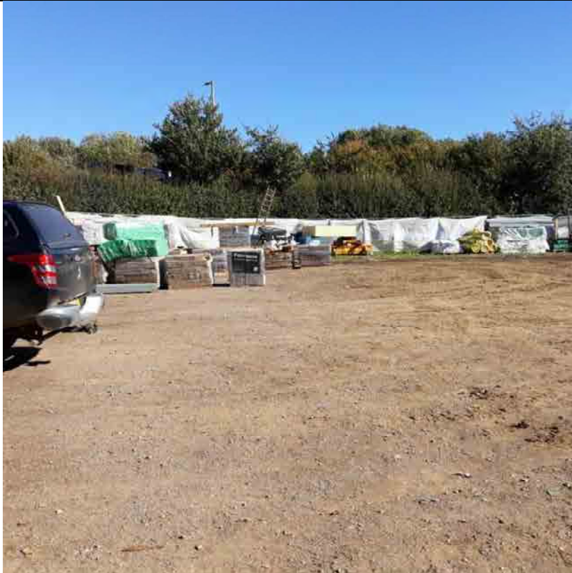
Photo 5: View inside the fenced storage area, looking SW to NE
