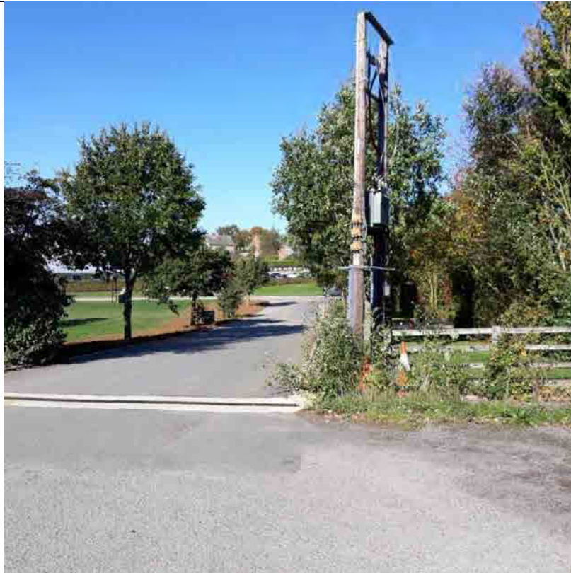
Photo 9: View of the electrical line running along the soft landscaped area in the southern part of the site
