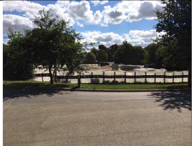
2. View SE from Cotefield Road to the works compound area at N end of Site.
