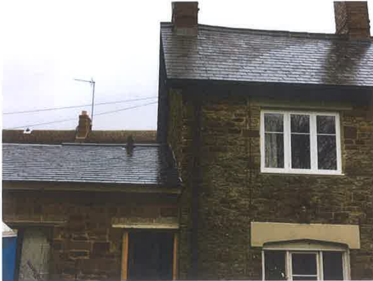
Slates In-situ (Lower Roof) against Existing House as of 28.11.19
