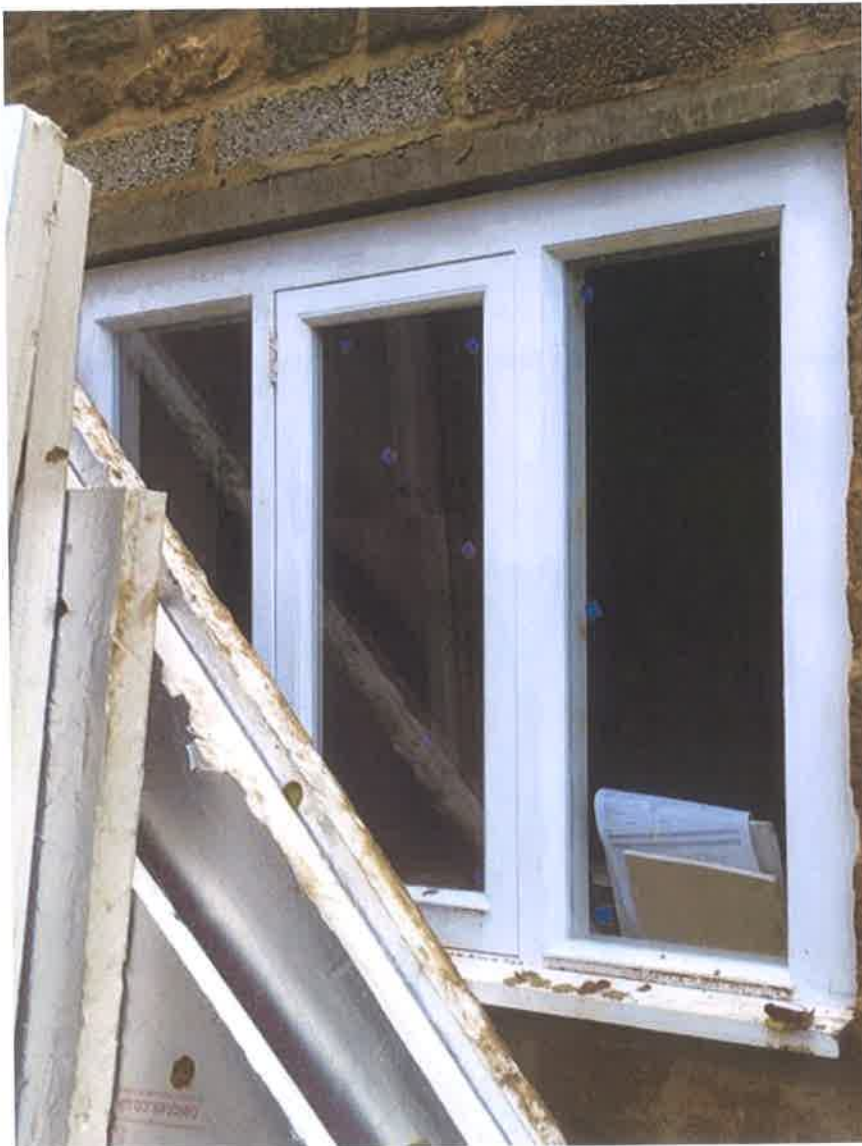
Timber Window to rear elevation in-situ 28.11.19
