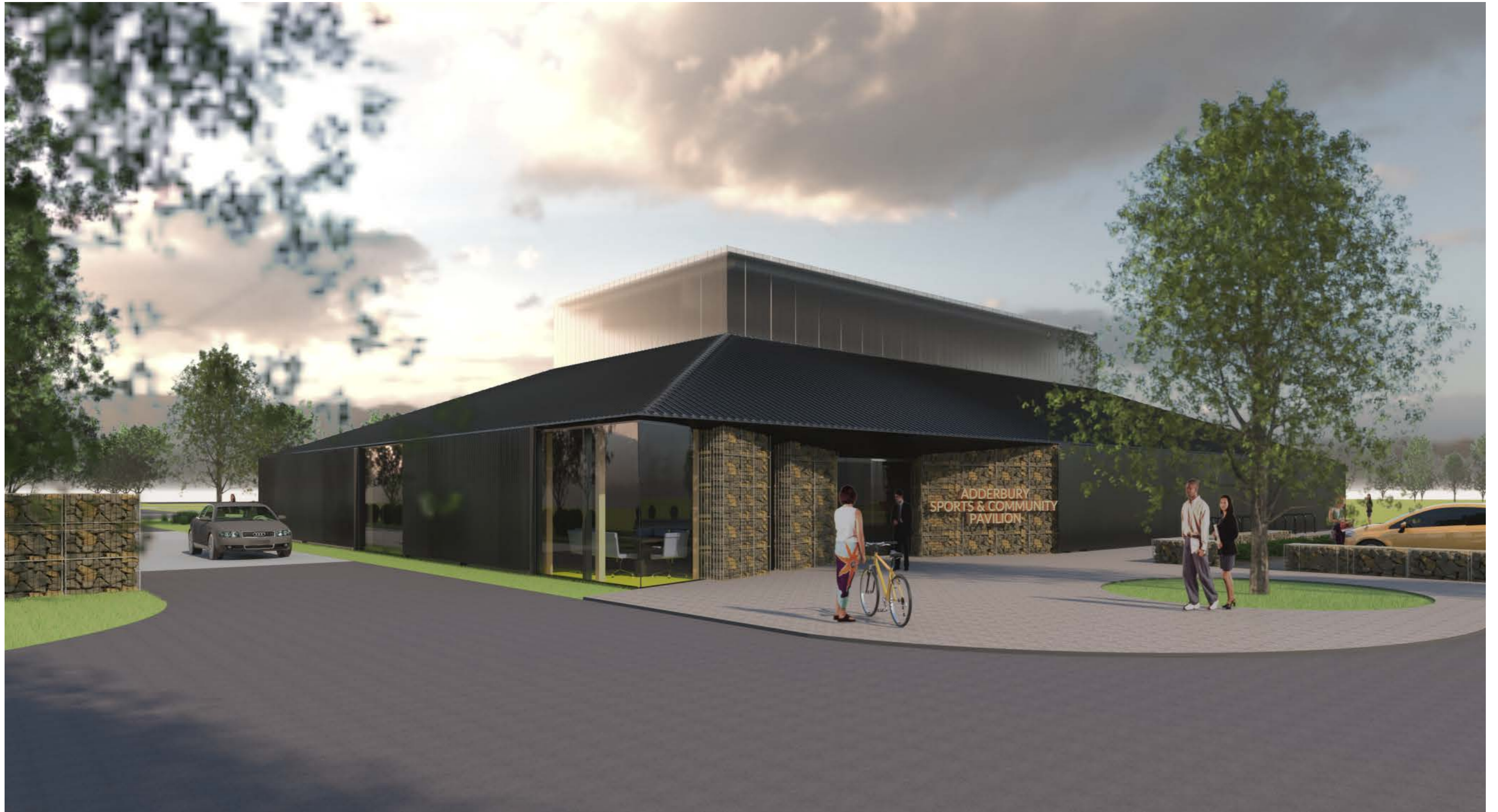
Fig 71: View from Milton Road showing local hornton stone in gabion baskets, used to frame entrance to new Pavilion
