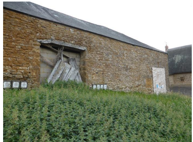
Blocked up opening
