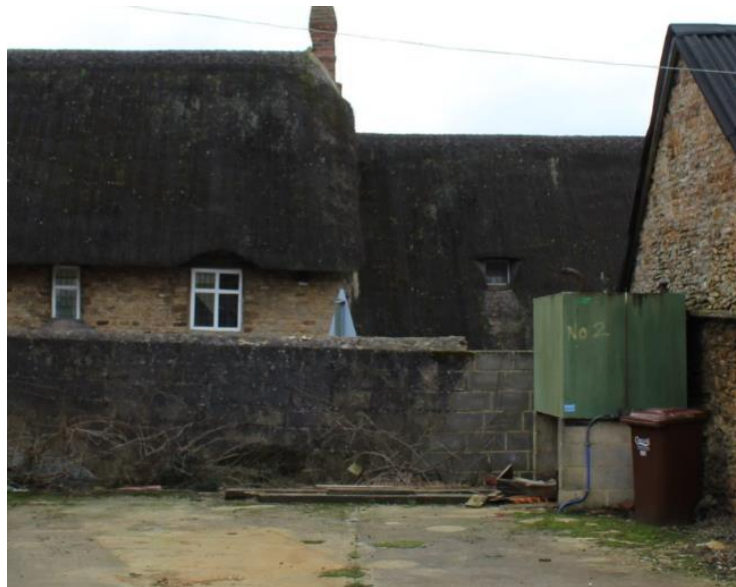
Photograph of wall to be removed showing blockwork construction
