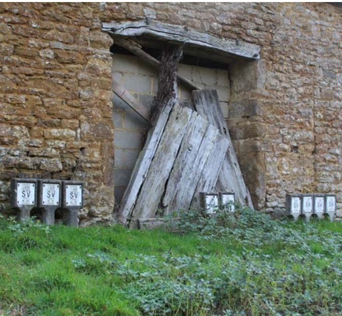
Fig. 27 - Inappropriate and substandard repairs
