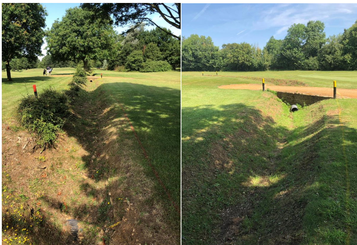
Figure 5-2: Site Drainage Ditches
