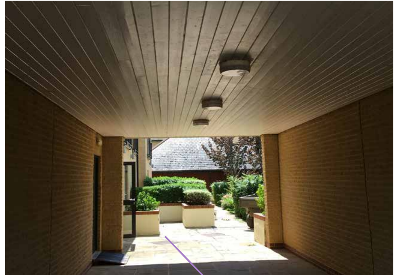
View of walkways near rooms Bicester Hotel Golf & Spa.
