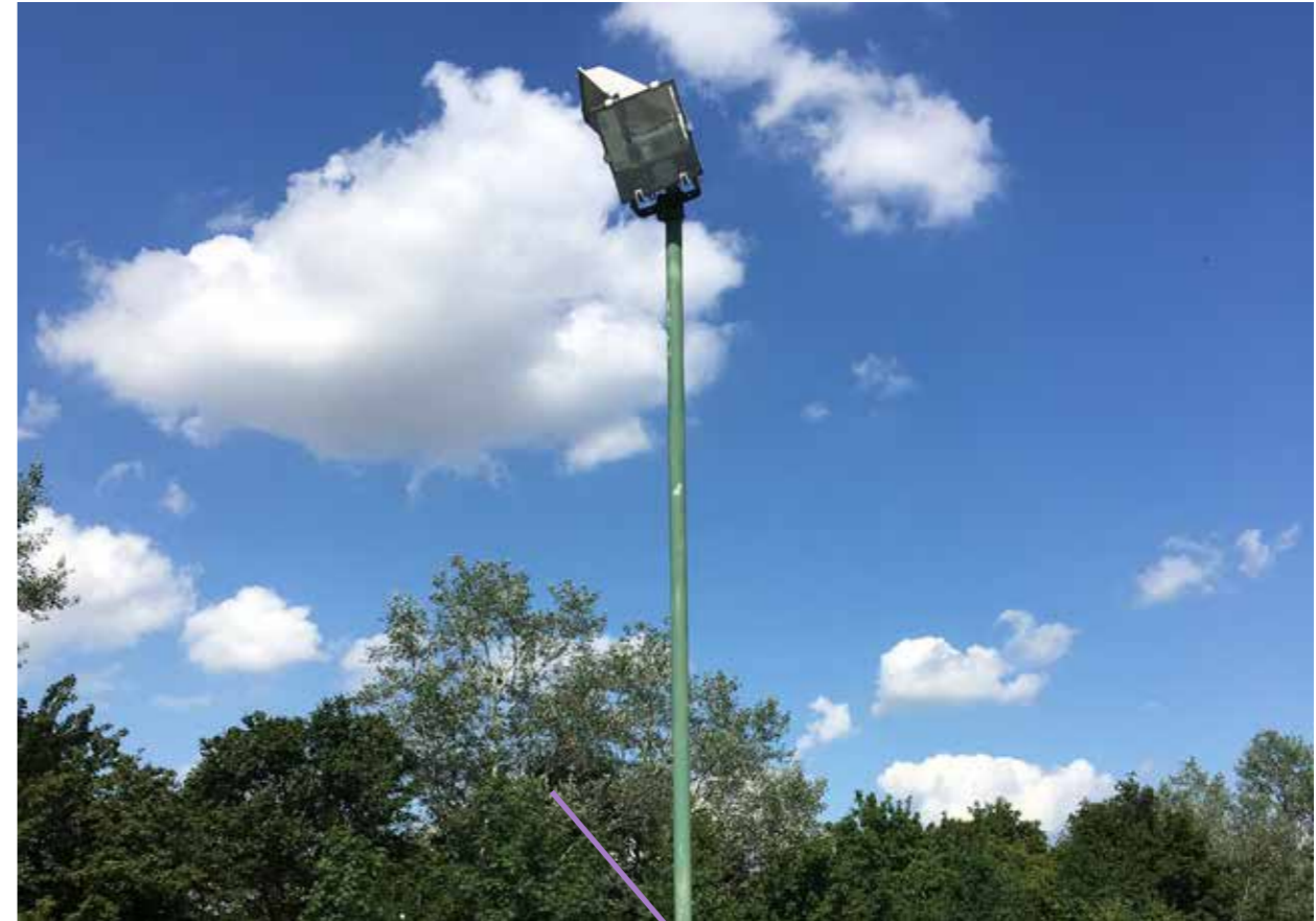
View of car park fitting near tennis courts Bicester Hotel Golf & Spa.
