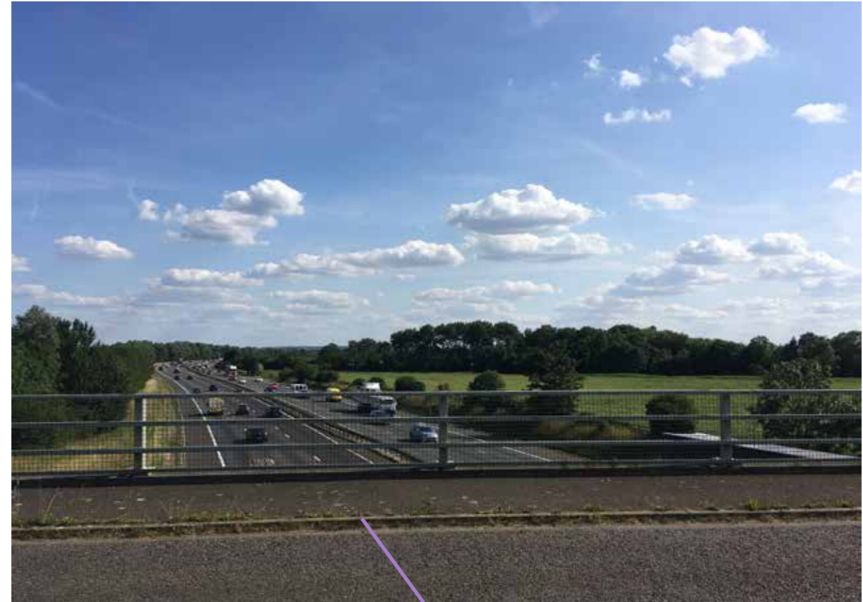
View from bridge on Green Lane over M40 looking south east.
