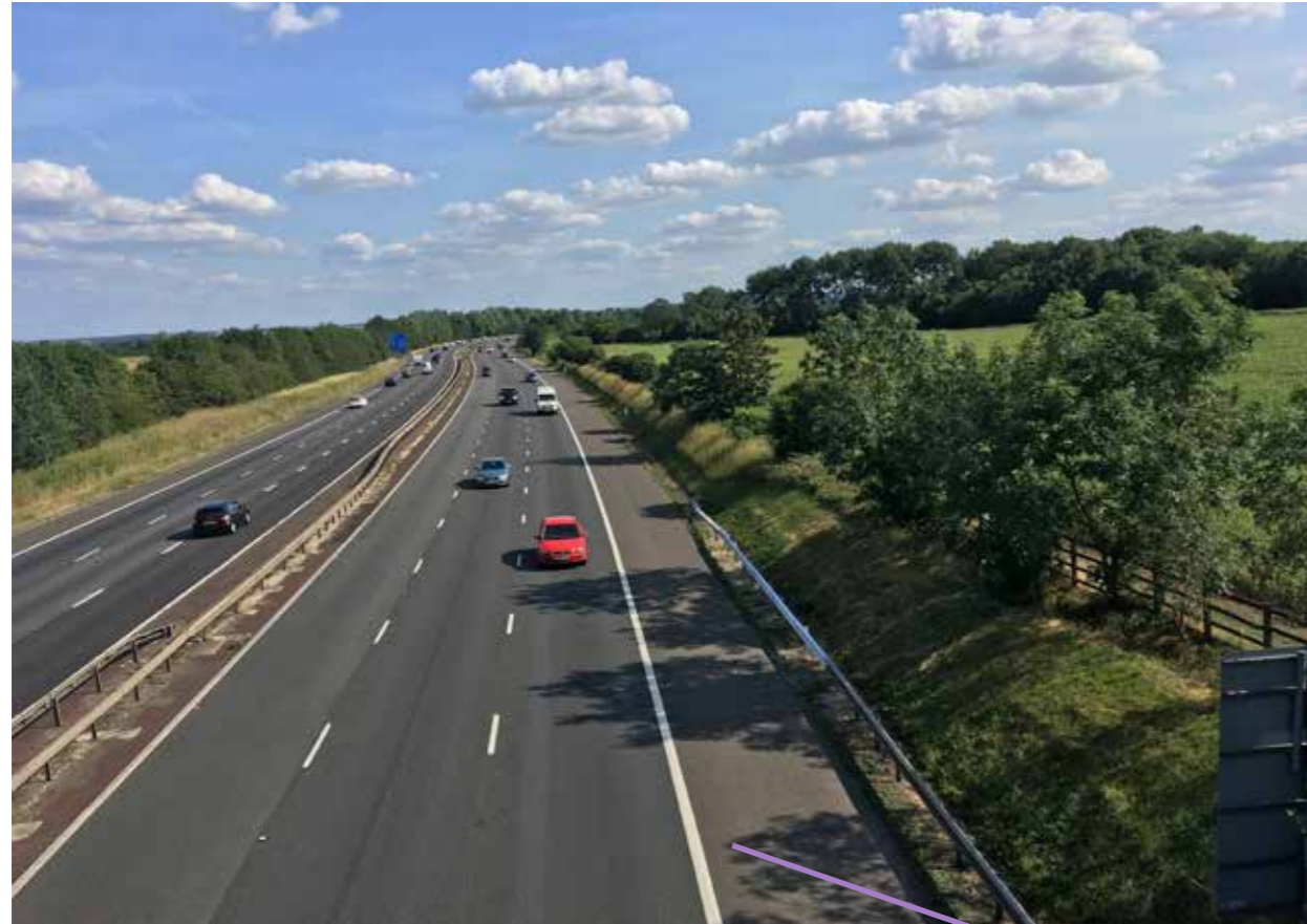
View from bridge on Green Lane over M40 looking south east, note footpath on right of photo.
