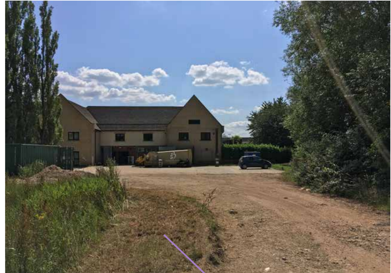
View of service yard Bicester Hotel Golf & Spa.
