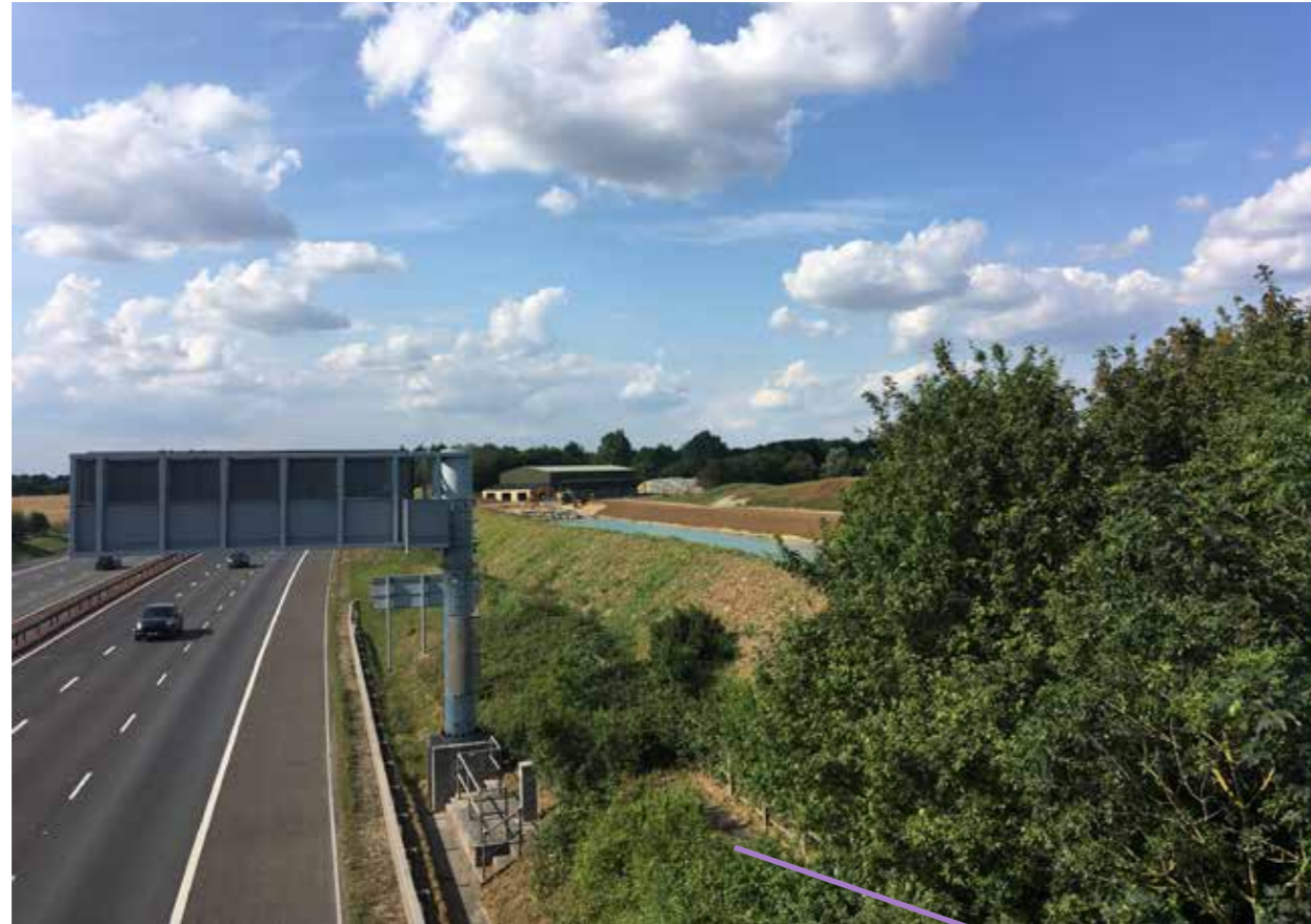
View from bridge on Green Lane over M40 looking north east.
