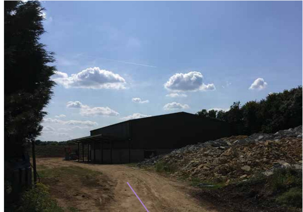
View of service area Bicester Hotel Golf & Spa.
