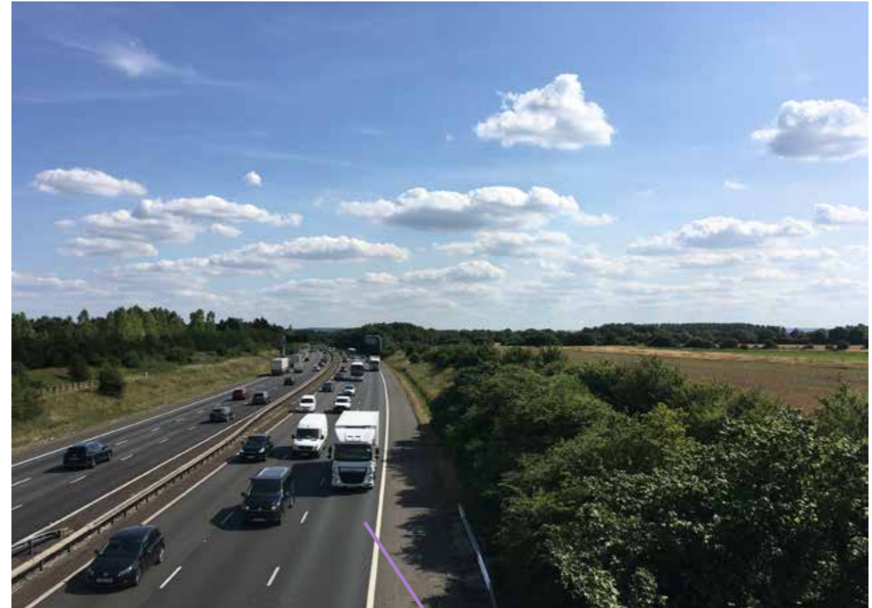
View from A4095 along M40 looking south east.
