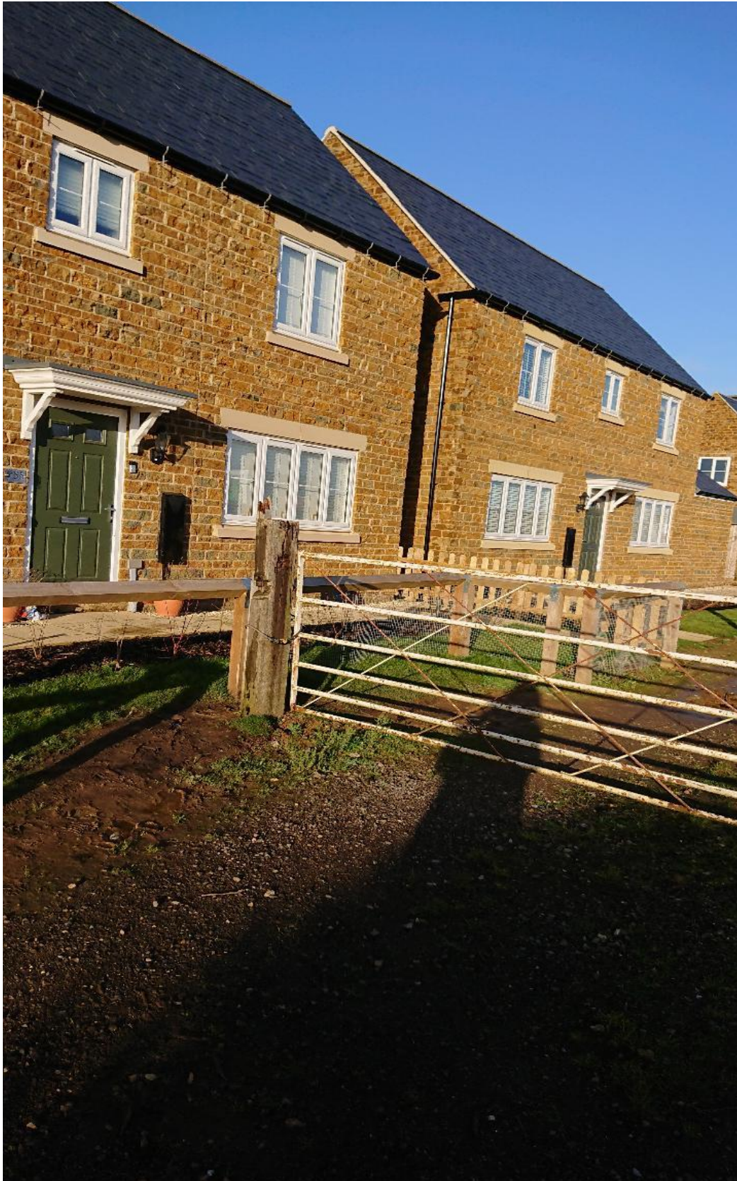
Pre-existing properties fronting Canal Lane with rear access for vehicles. Planning documents do not mention Right of Way gate.
