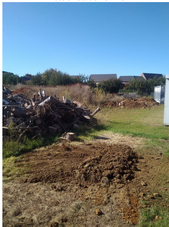
Plate 10 Location of TP3 near stockpiled material
