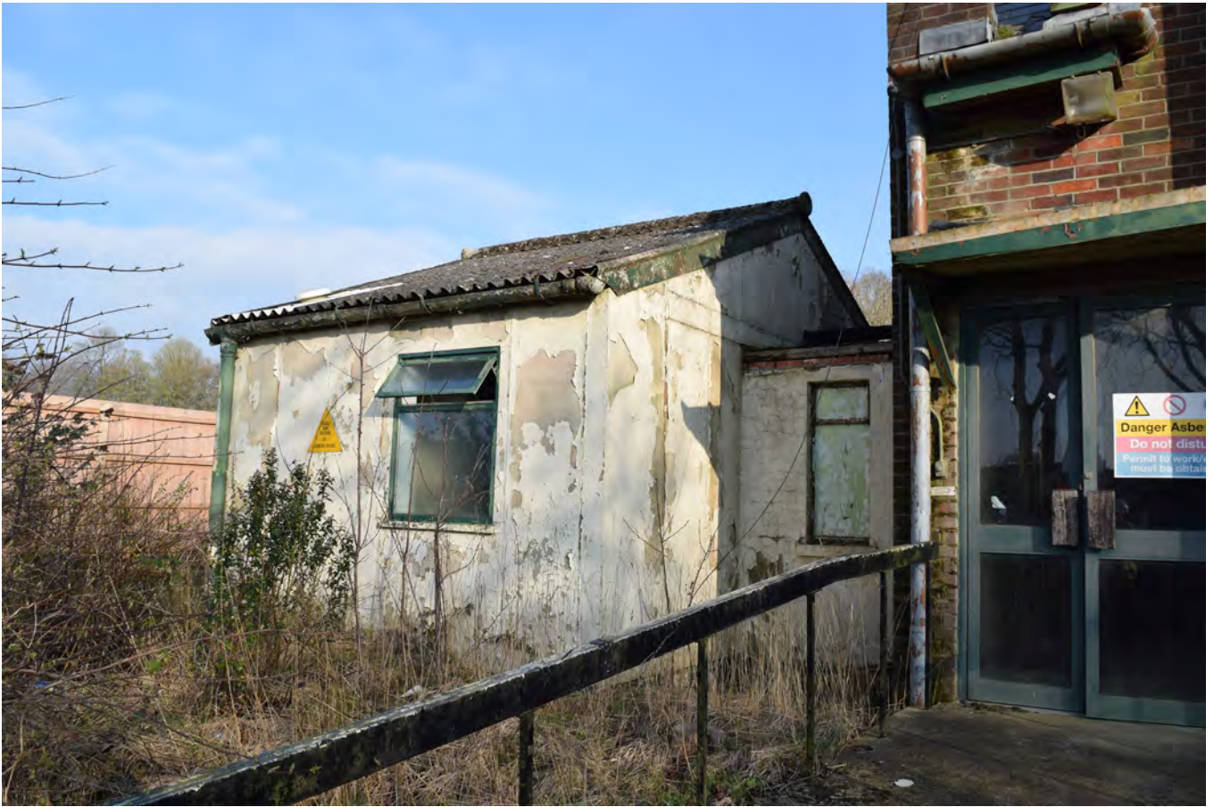
Plate 457.3 View of concrete wc extension
