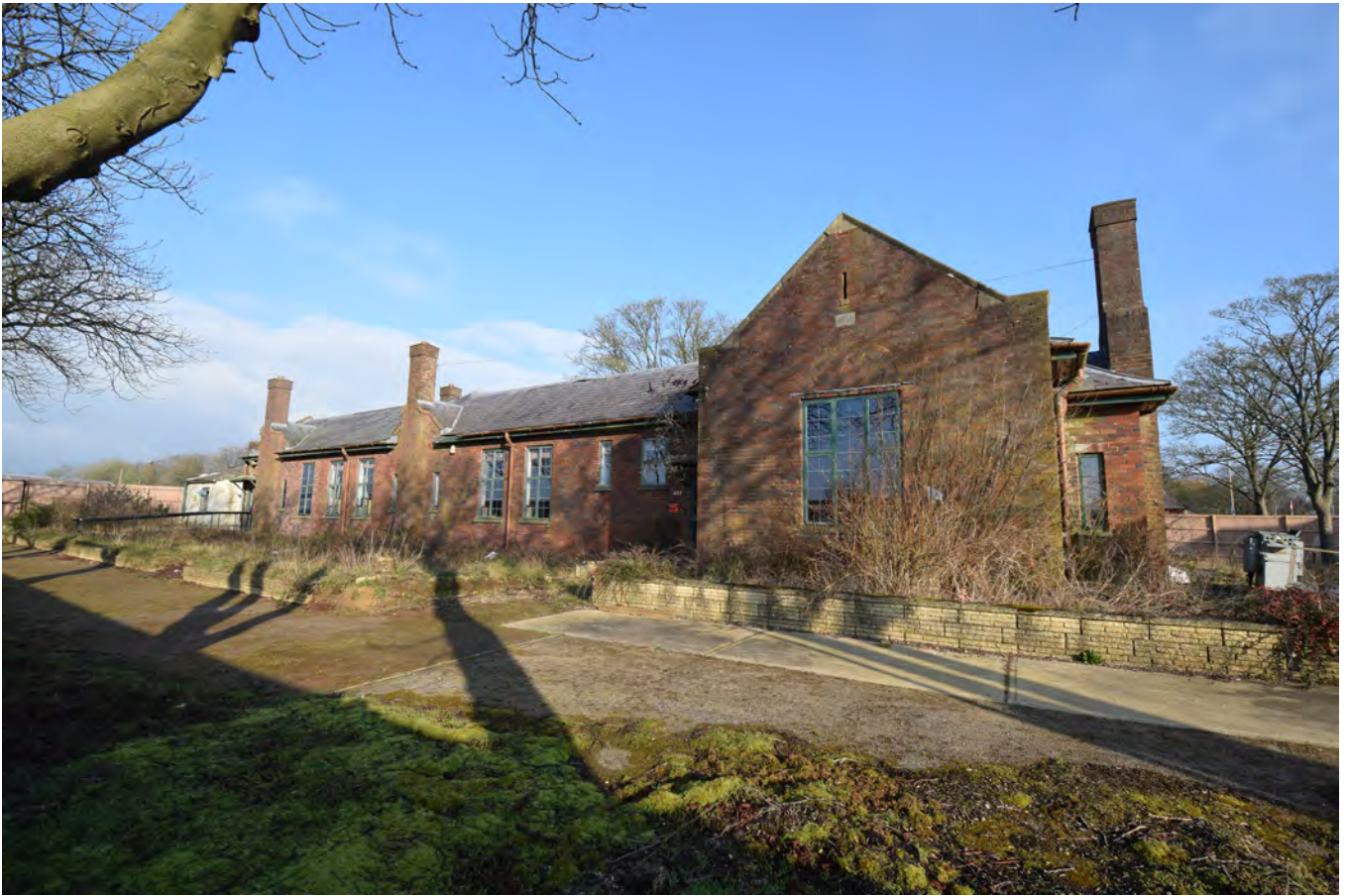
Plate 457.1 View of front (north) elevation
