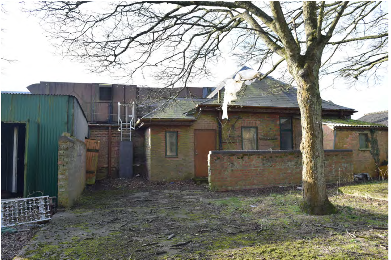
Plate 457.5 View of south elevation, central section
