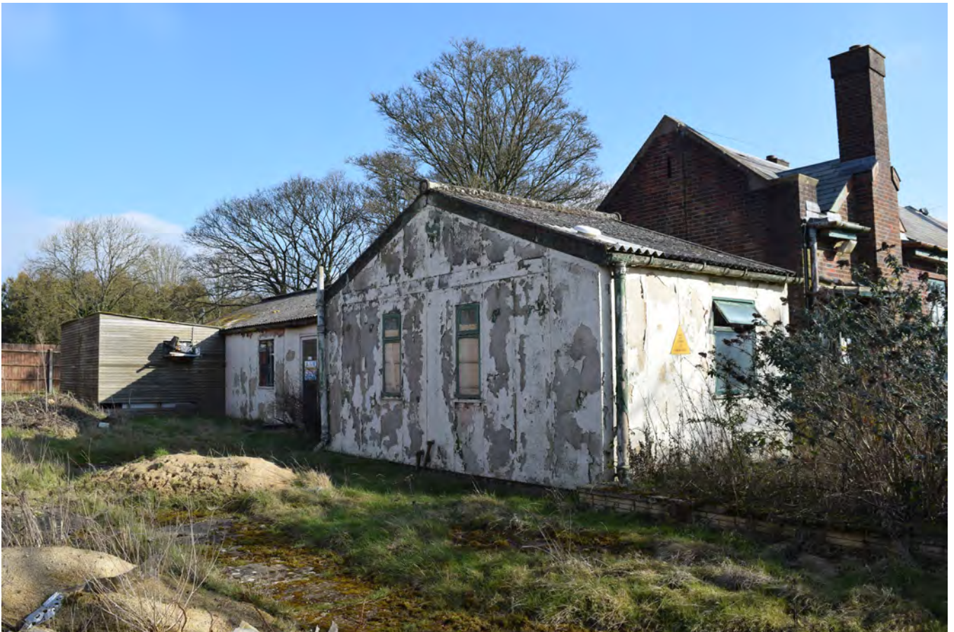
Plate 457.8 View of east elevation
