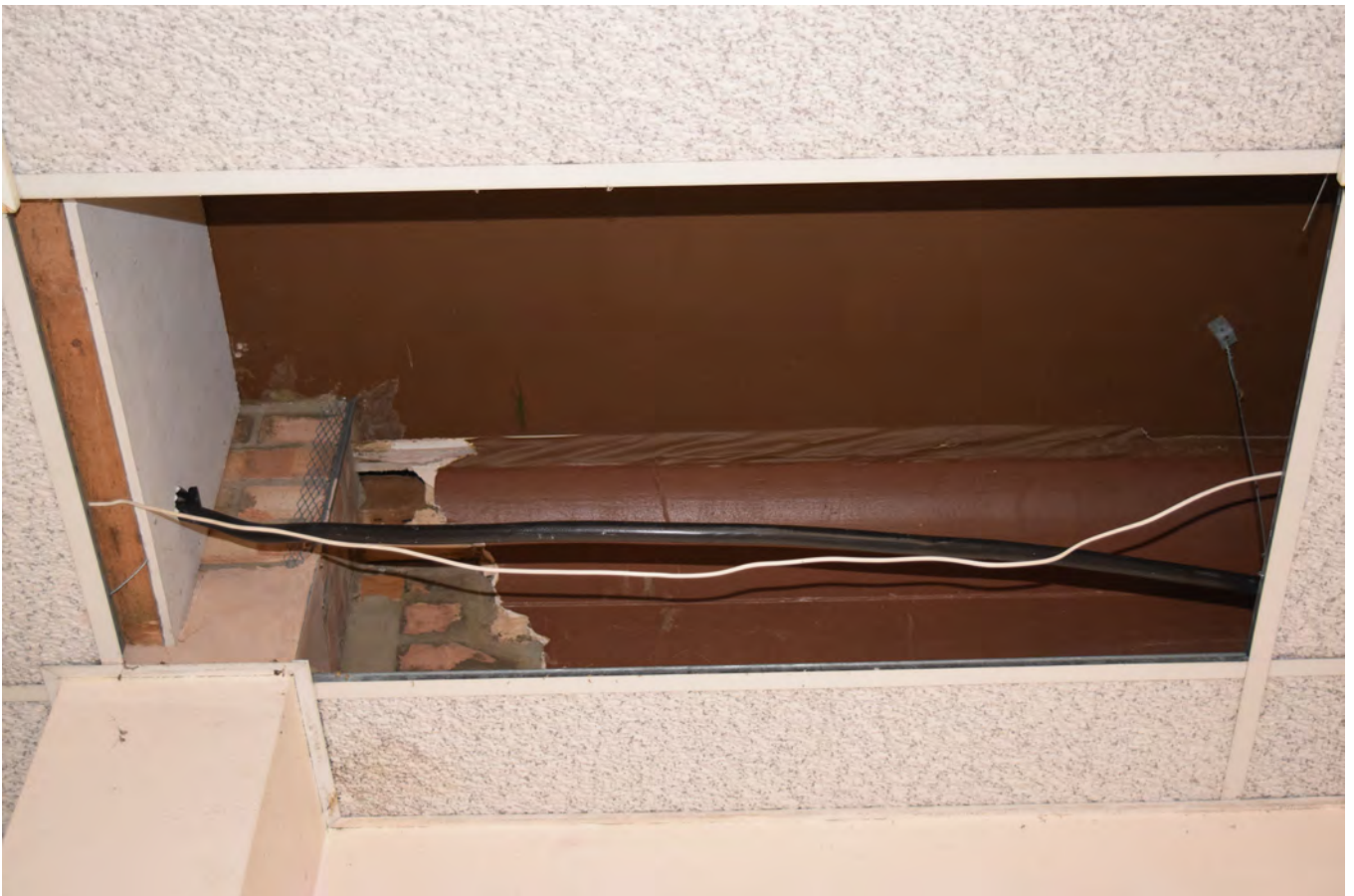
Plate 457.18 Detail of former ceiling within main dining area
