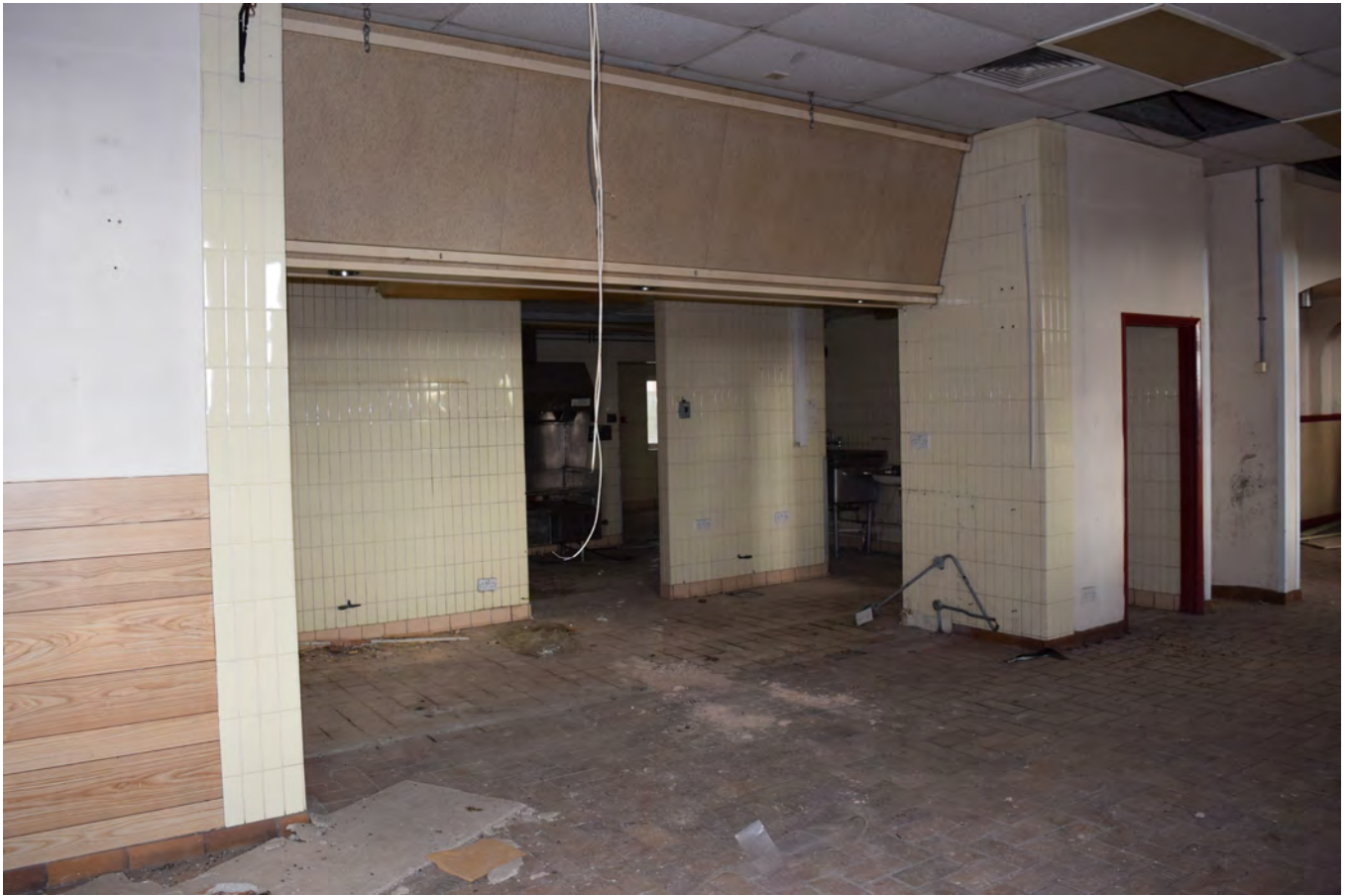
Plate 457.19 Detail of servery and entrance to kitchens
