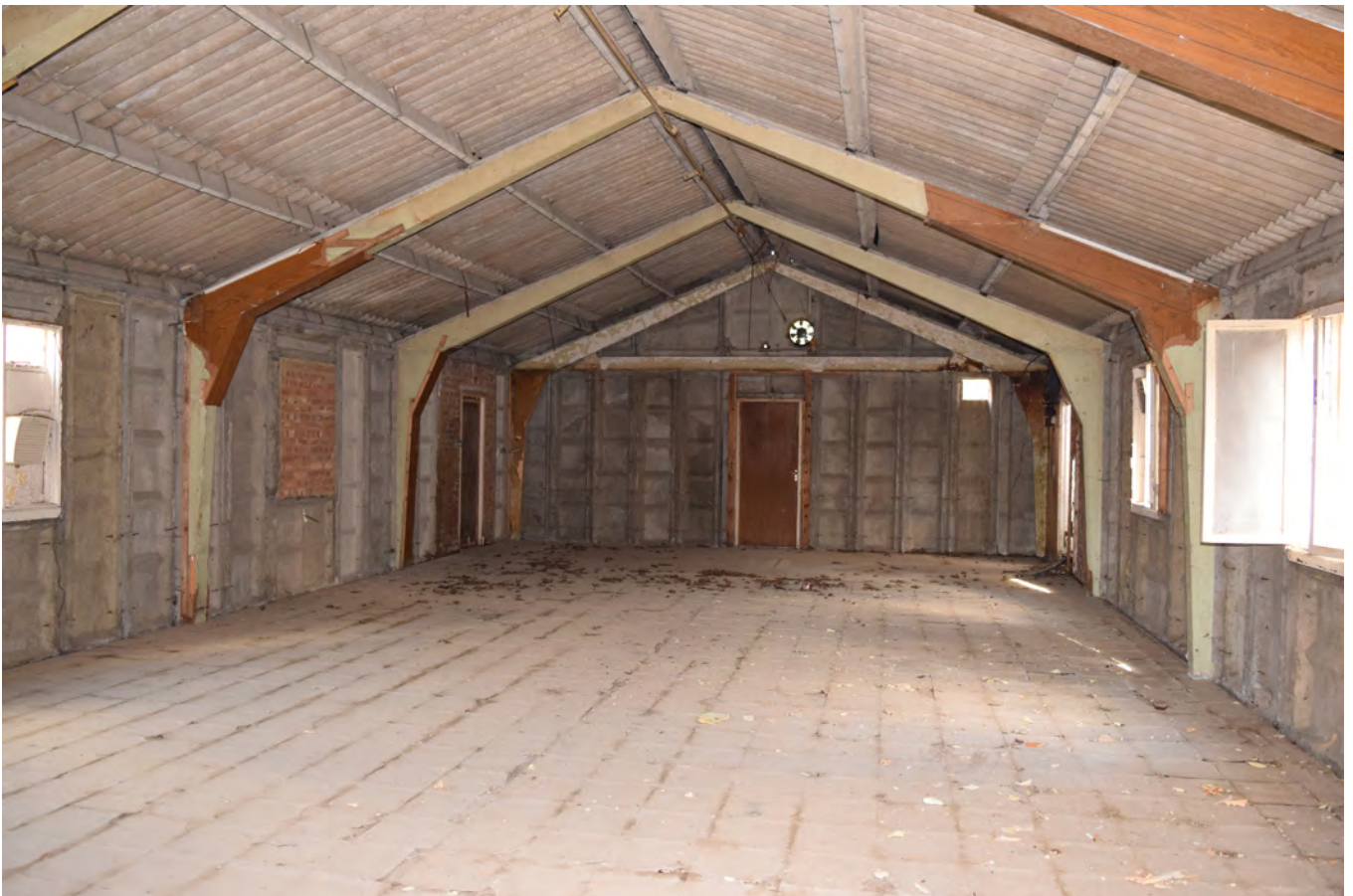
Plate 457.12 View of large concrete extension interior
