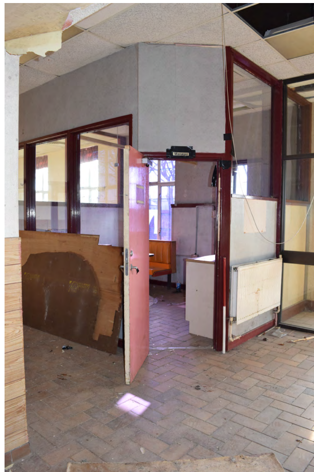
Plate 457.14 View of games room within entrance lobby
