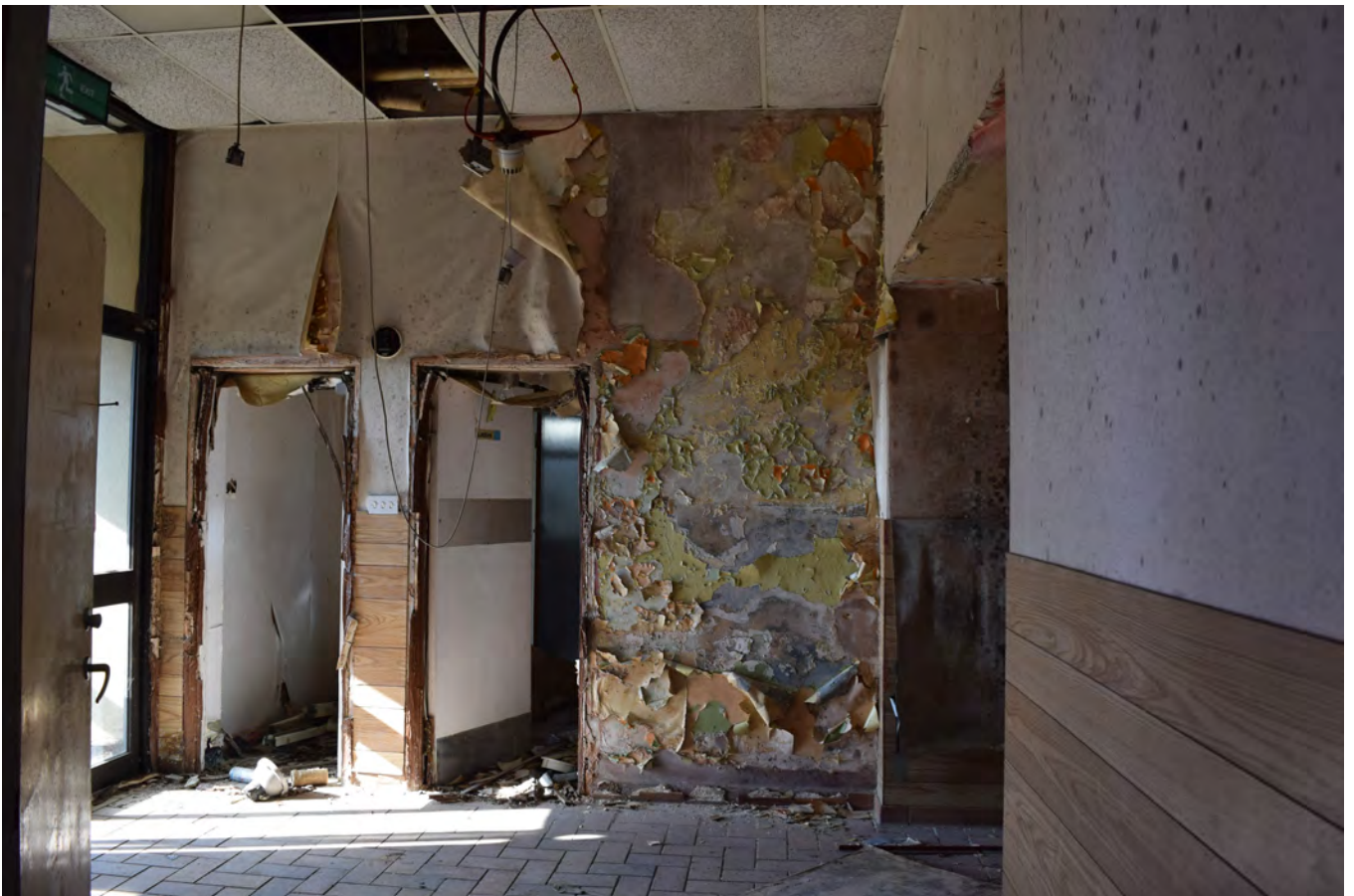
Plate 457.10 View of entrance lobby towards wc extension
