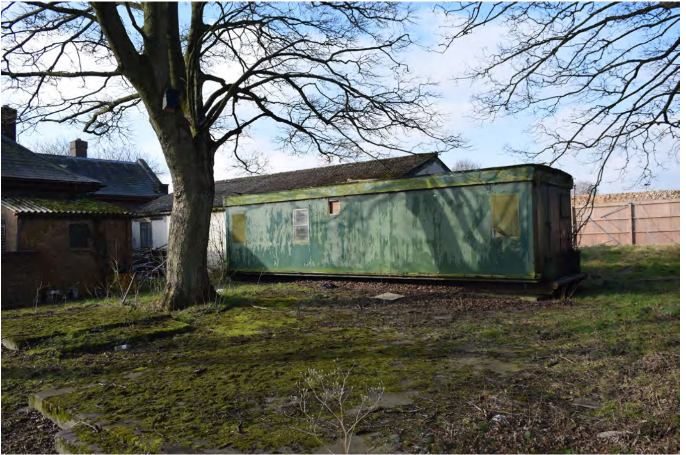
Plate 457.9 View of porta cabin extension
