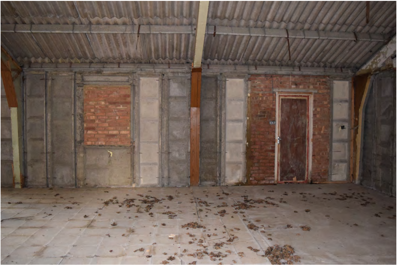
Plate 457.13 Detail of blocked openings within large concrete extension
