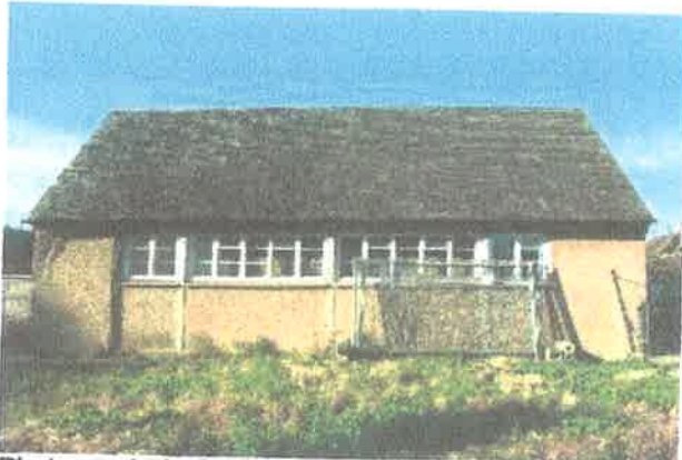
Photograph 1. St George's Church viewed from the east.
