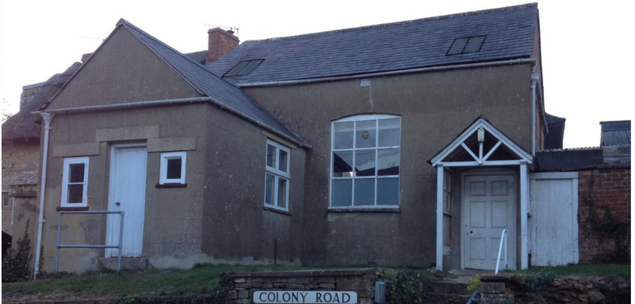
Photograph of East elevation showing proposed Velux roof windows to be installed in existing slated roof
