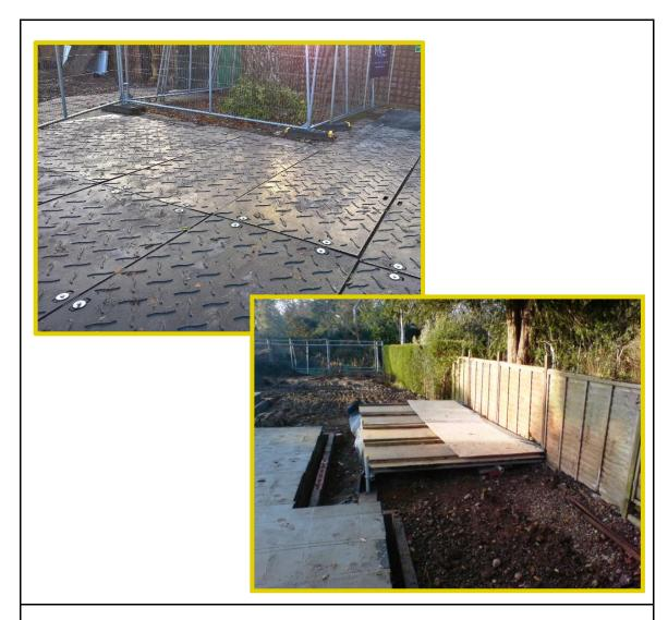
New temporary ground protection should be capable of supporting any traffic entering or using the site without being distorted or causing compaction of underlying soil.
