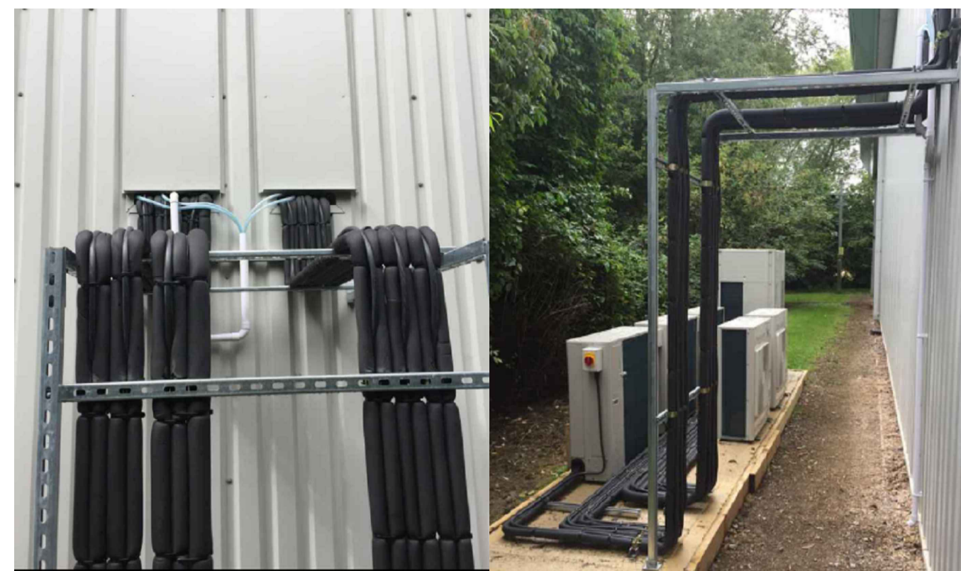
Example of the type of bridging frame that will be used.
