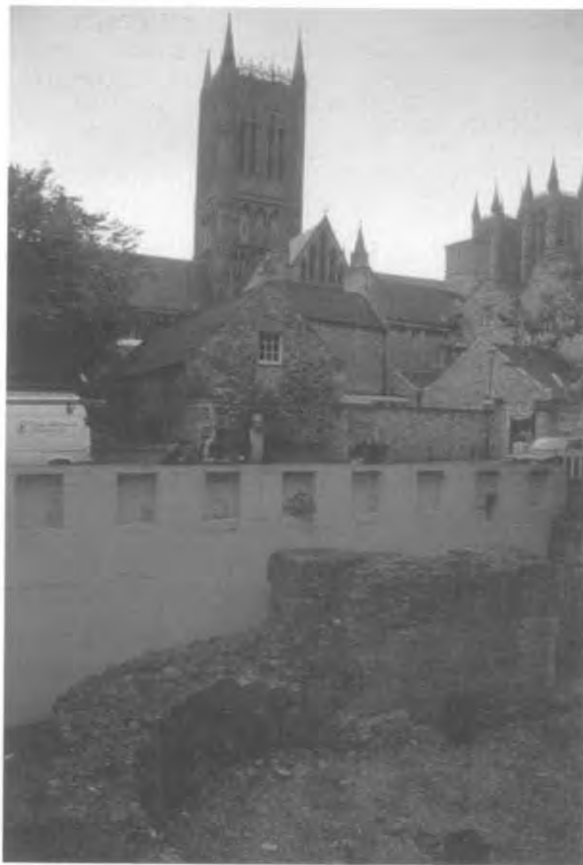
Fig. 8: Roman towns of rectangular plan often, even if not always, overlie Roman forts or fortresses. Sometimes, such as here at Lincoln, the civilian-period stone wall and gate are directly superimposed over its military timber predecessor; sometimes the position has shifted by a few metres.
