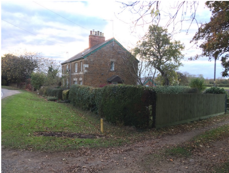
Plate 2: Nos. 11 and 12 South Newington Road, view to south
