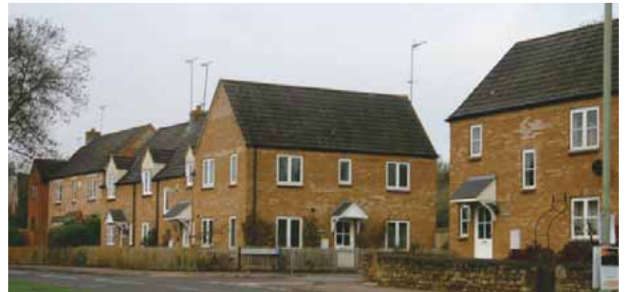
Housing developments of the later 20 th Century exhibit a wider spectrum of construction materials, including buff/yellow brick and painted stonework.
