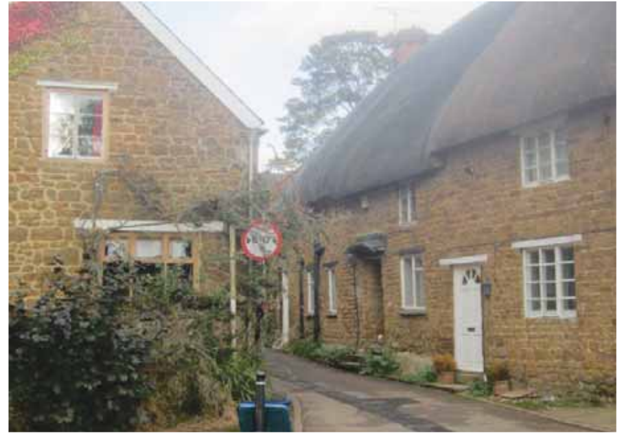
Buildings within Bloxham's historic core are generally constructed of locally quarried ironstone, with detailed stonework over doors and windows on principal elevations.
