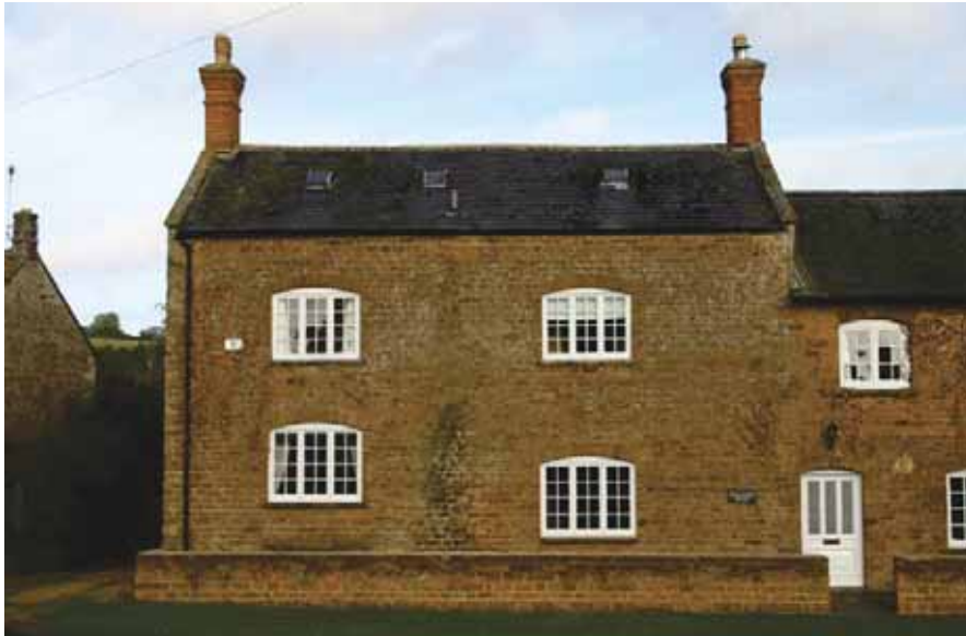
Traditional building materials within the historic village core include dressed or coursed ironstone.
