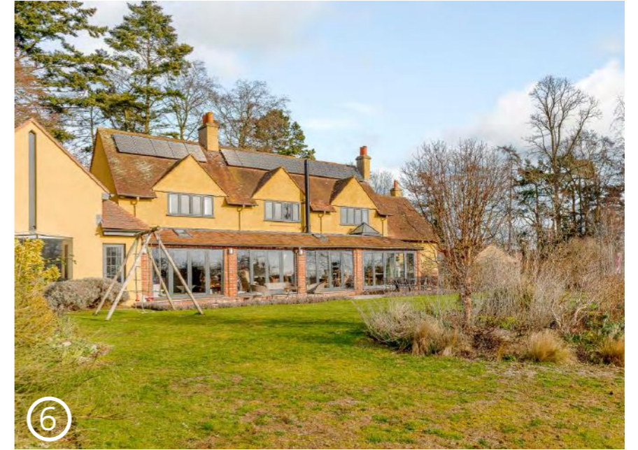
Existing Dwelling House
