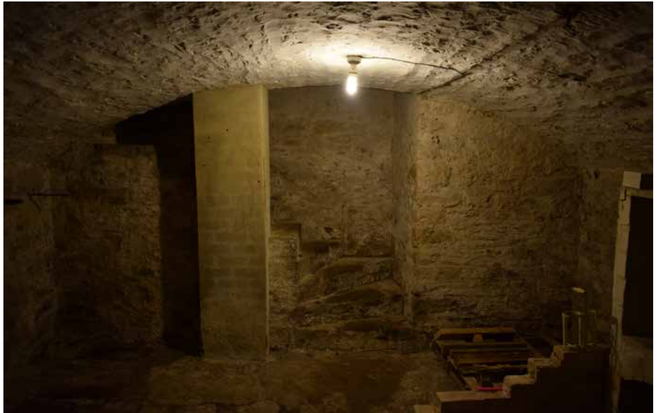
Fig 33: Cellar showing the steps located under the stair case
