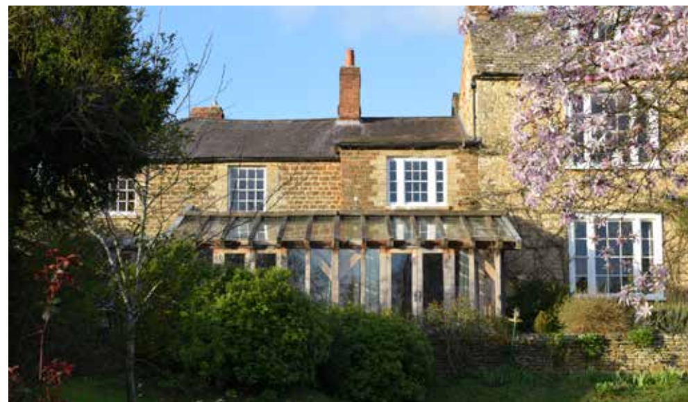
Fig 24: View of the rear (south) elevation of the former service wing showing the 8 over 8 sash windows to the first floor
