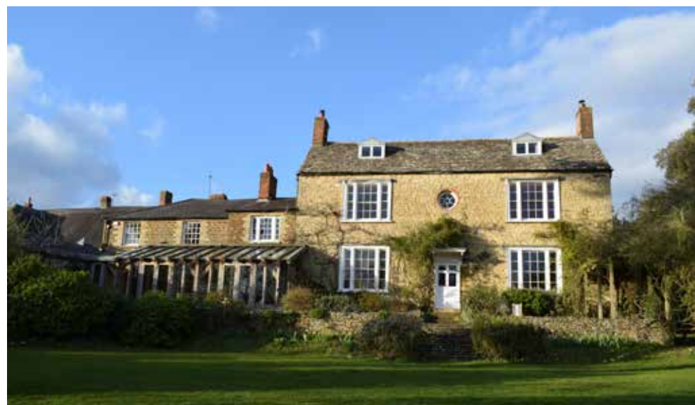
Fig 21: Rear (south) elevation of the house with symmetrical elevation and former service wing to the west with new conservatory and reintroduced dormers to the roof.
