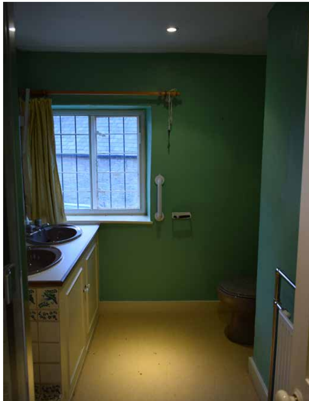
Fig A3.6: Bathroom in the former service wing to be enlarged by relocating modern cylinder heater and enclosure and moving the approved partition.
