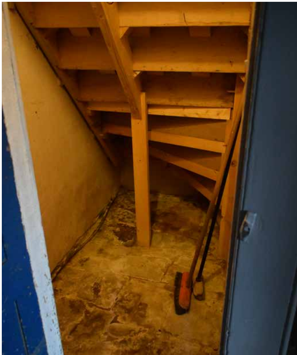
Fig A3.1 & A3.2: The stair in the service wing which appears to have been recently replaced. Proposal is to remove and install a new, compliant stair in this location
