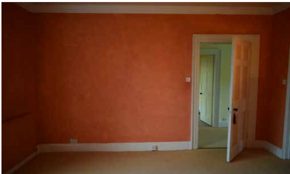
Fig 35: The wall between the bedroom and the hall landing mirroring the other bedroom. Clear evidence from the skirting board that there was a previous matching opening in this wall, since blocked
