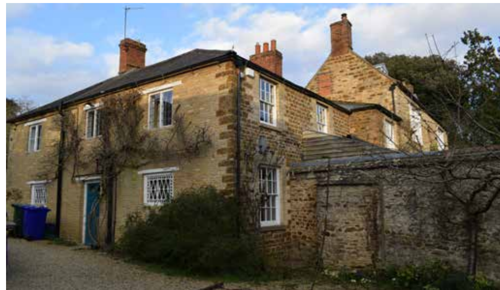
Fig 23: View of the former service wing from the south west showing the symmetrical west elevation of the north south range with the wrought iron casement windows, and the rear (south) elevation with sash windows and the lean-to extension, and the roof of the conservatory over the wall running south west from the elevation.
