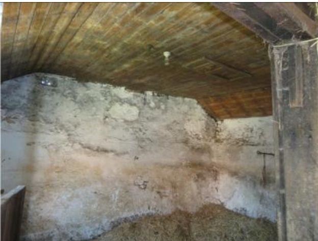
Photograph 21. Example of a bay within Building 3
