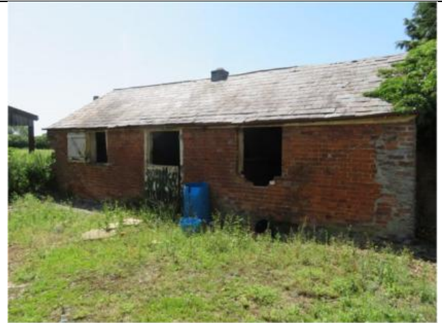
Photograph 16. The north-east elevation of Building 3
