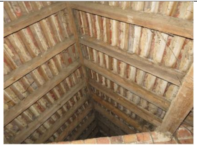
Photograph 10. Example of the underside of the roof in Building 1
