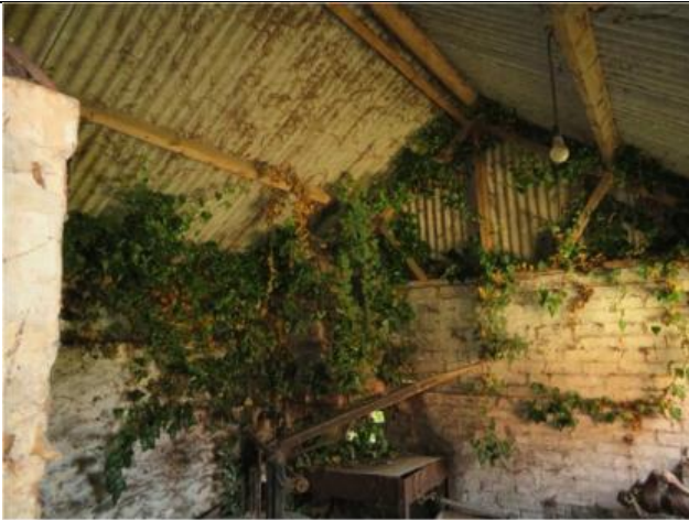
Photograph 15. The interior of south-western part of Building 2
