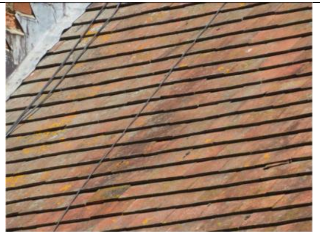
Photograph 4. Example of the tiles on the roof of Building 1
