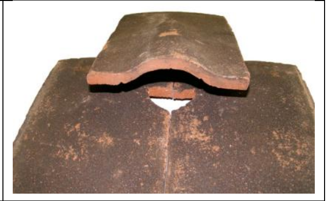
Photograph 26. Example of bat access tile
