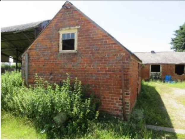
Photograph 13. The north-east elevation of Building 2
