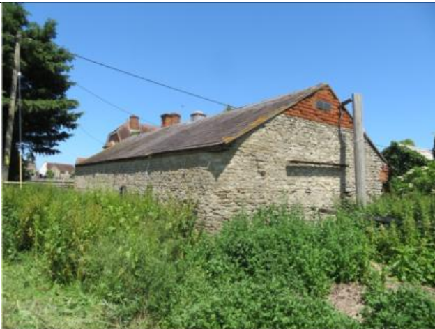
Photograph 17. The south-west and south-east elevations of Building 3
