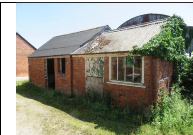
Photograph 11. The north-west and south-west elevations of Building 1
