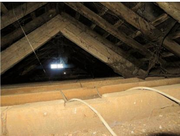
Photograph 23. The enclosed roof void within Building 3 (view to south-east)
