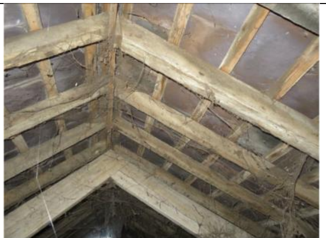
Photograph 24. The underside of the roof within Building 3
