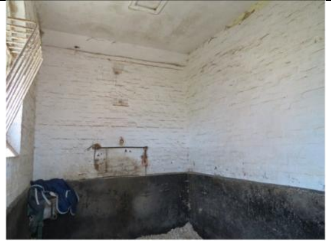
Photograph 8. Example of one of the bays in Building 1
