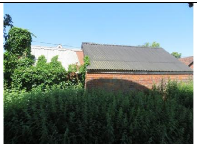
Photograph 12. The south-east elevation of Building 2
