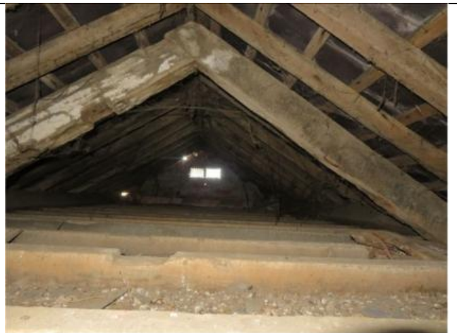
Photograph 22. The enclosed roof void within Building 3 (view to north-west)
