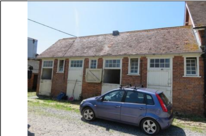
Photograph 1. The north -east elevation of Building 1
