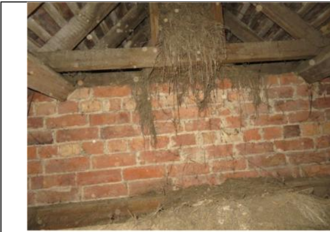
Photograph 9. Part of the enclosed roof void within Building 1
