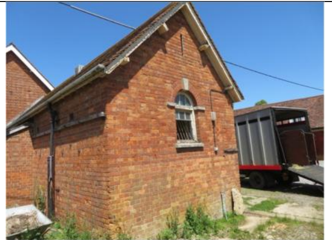
Photograph 2. The south-east elevation of Building 1
