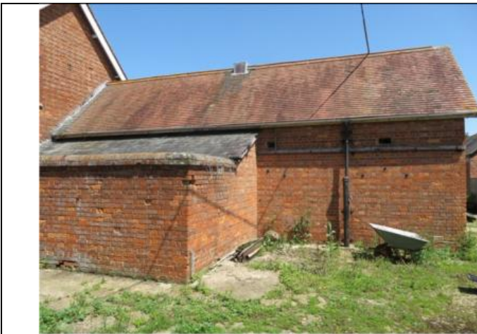
Photograph 3. The south-west elevation of Building 1
