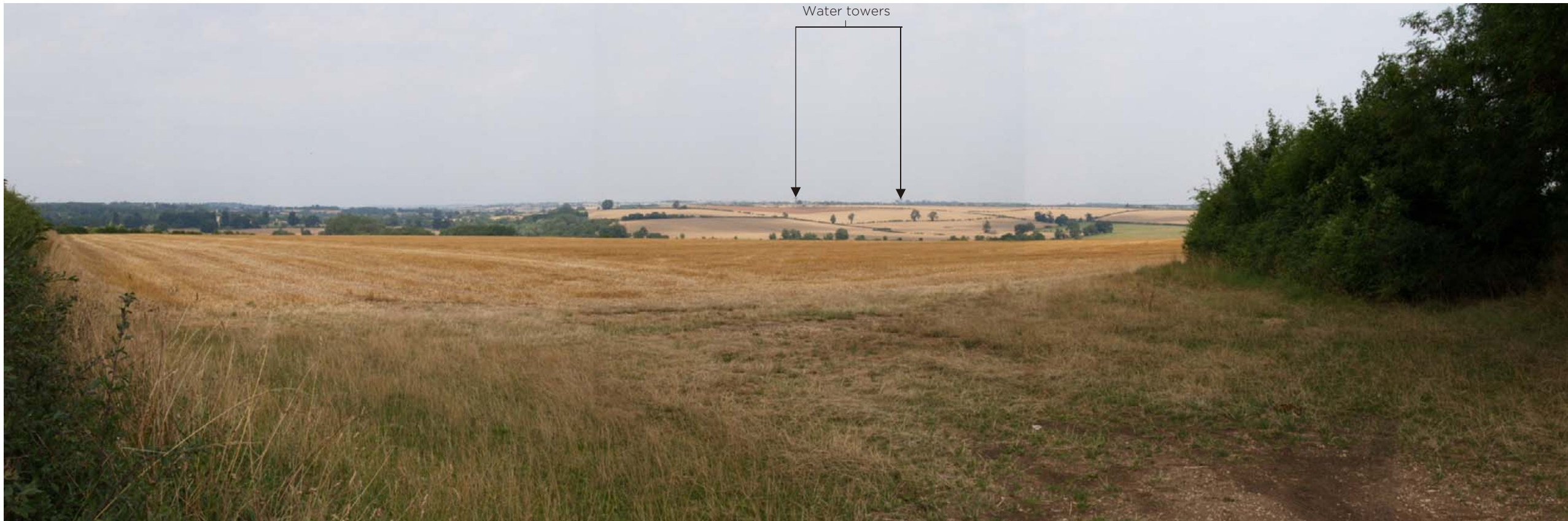
Viewpoint 9: From A4260 turning towards Tackley Village, water towers visible on skyline (see inset on Plan L2)
