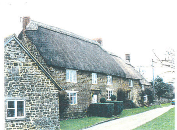
Vernacular Architecture - building materials accurately reflect the complex underlying geology of the District landscape, as in the case of these cottages on the western ironstone.
