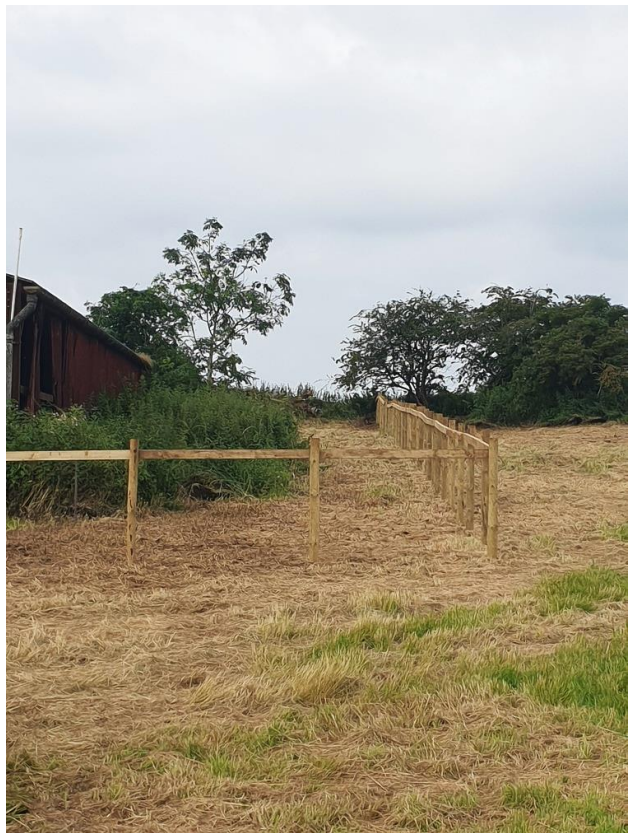
Figure 3 – Fencing on site (north)
