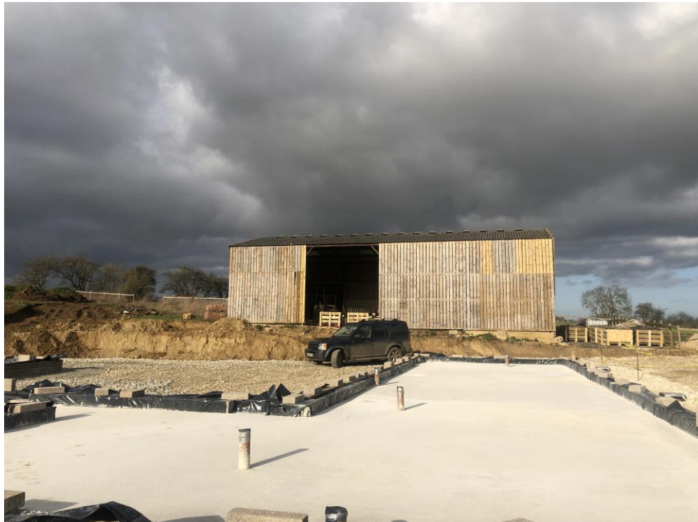
Figure 2 – Barn to be Converted (South Elevation)
