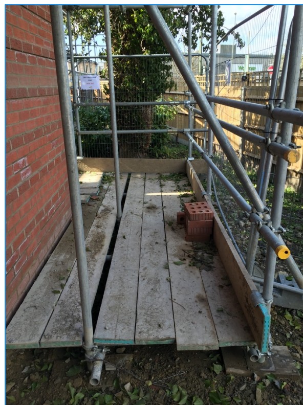
Scaffold ground protection
