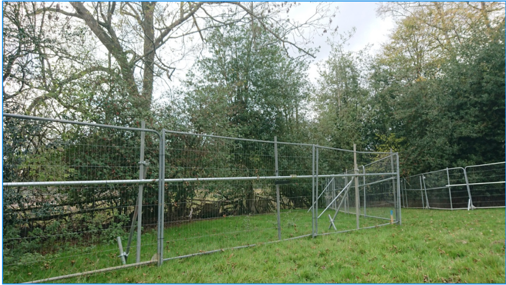
Typical tree protection barrier construction
