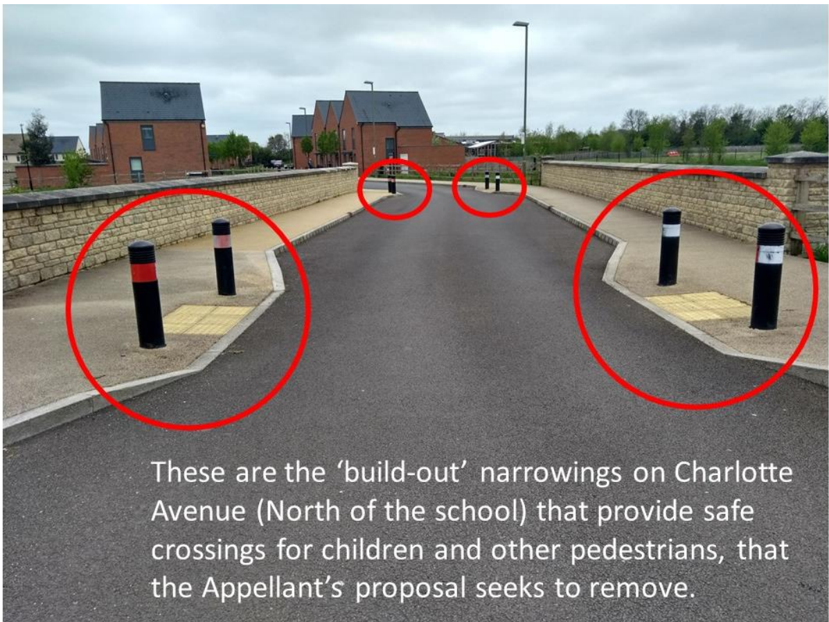
Figure 2-3: Photo showing the build-out narrowings on the mid-Phase 2 Charlotte Avenue bridge to the north of Gagle Brook Primary school; children from Phases 3-4 plus the south side of Phase 2 beyond this point use these as they are the only safe crossings to the north (school) side.
