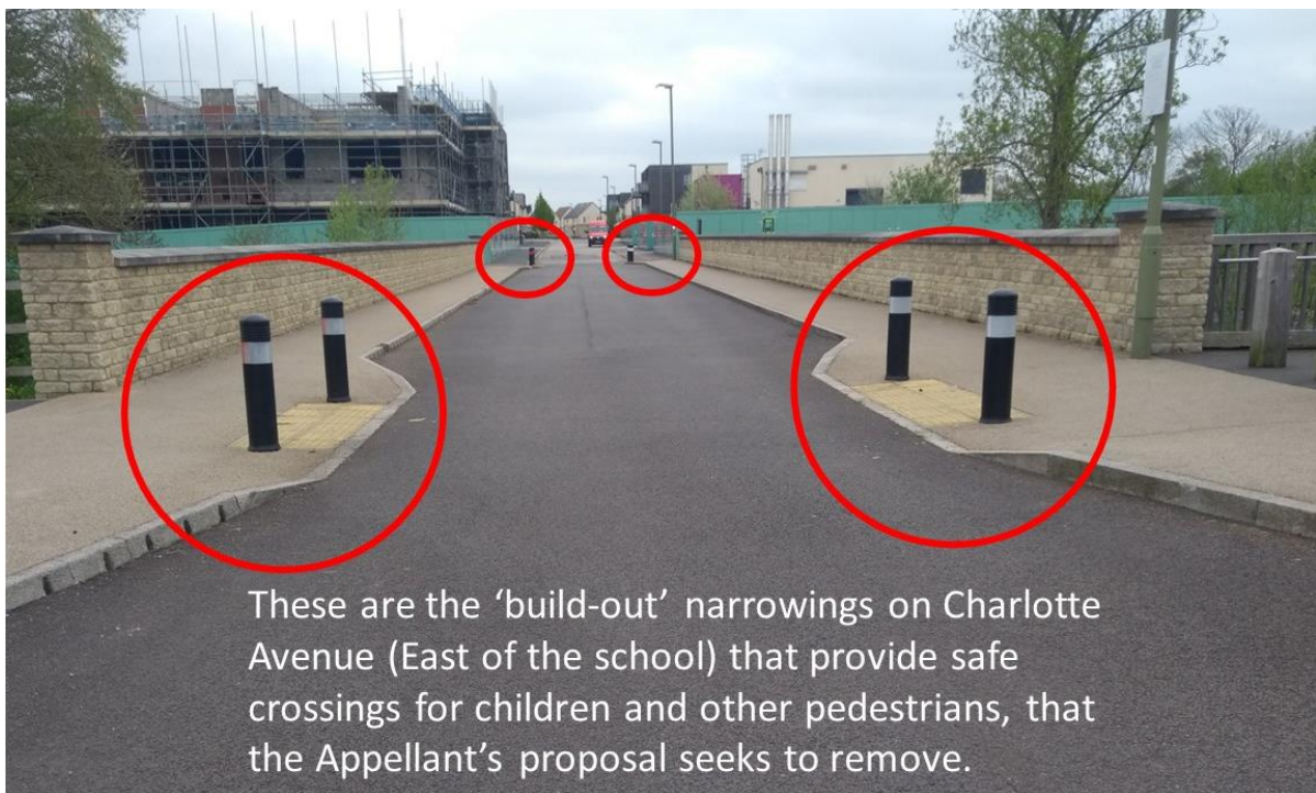
Figure 2-5: Photo showing the build-out narrowings on the Charlotte Avenue bridge to the east of Gagle Brook Primary School, with the Community Hub (under construction) and Eco Business Centre on the left side (as viewed here, facing east), and Local Centre (not built) and Energy Centre (right).
