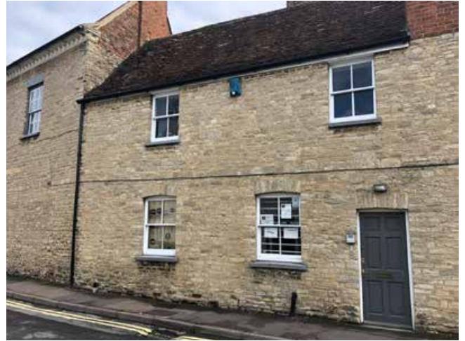
Simple yellow stone façades with lintel detailing
