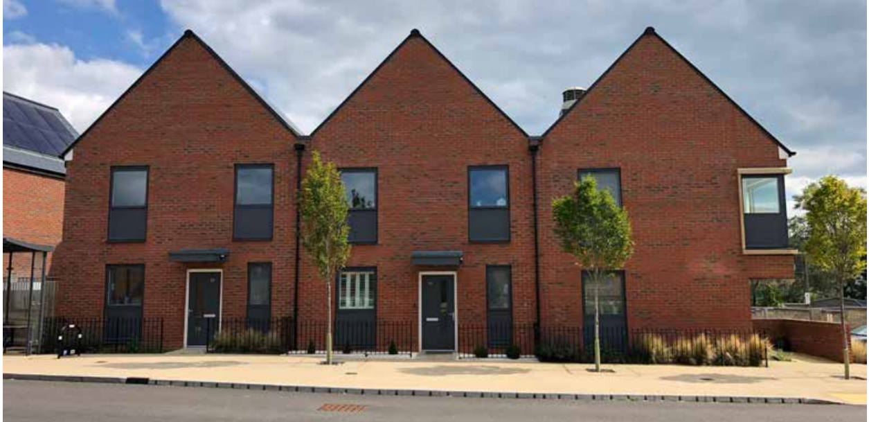
Terraces at the Exemplar Site
