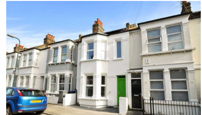
Hiley Road – A Victorian Terraced house retrofitted to achieve Passivhaus certification with a space heating demand of just 15kWh/m 2 , Located in Kensal Green, London
