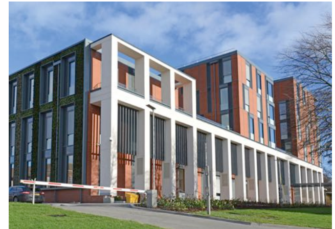
University of Leicester Centre for Medicine – This 13,000m 2 building has a 300 seat lecture theatre, laboratories and teaching spaces. It is Passivhaus certified with a primary energy use of just 116kWh/m 2 .
