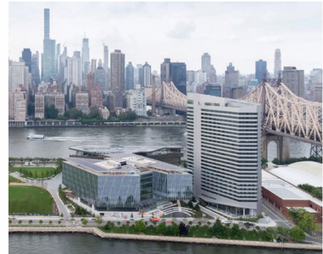
The House, Cornell Tech, USA - Passivhaus certified 26 storey student accommodation with 352 units
