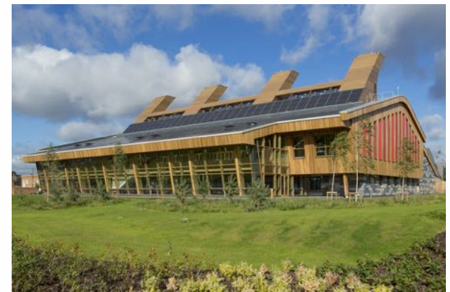
University of Nottingham GSK Laboratory for Sustainable Chemistry – This 4,200m 2 building contains laboratories and general teaching spaces. It is BREEAM Outstanding and LEED Platinum.
