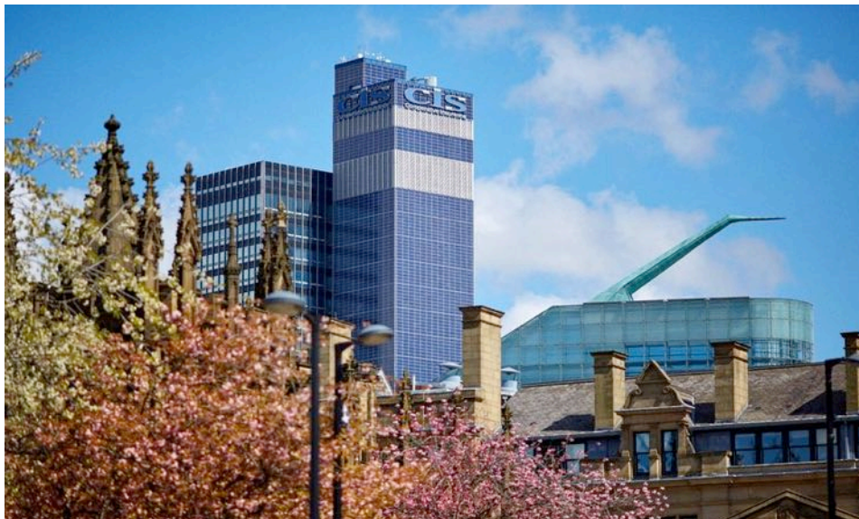
Figure 2.5 - With 576kW of solar photovoltaic panels installed, the CIS tower in Manchester was Europe's largest vertical solar array when completed in 2006.
