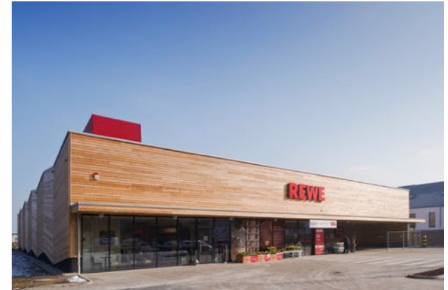
REWE Supermarket – The first Passivhaus supermarket in Germany was created in 2014 in Hanover. It has a space heat demand of just 12kWh/m 2 /yr and uses 30% less energy than a conventional supermarket. ©PassREg
