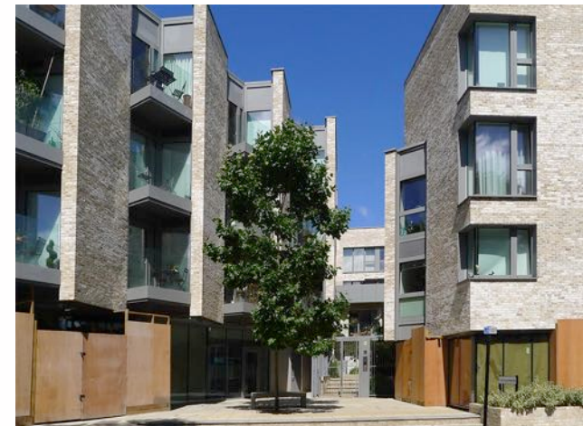
Chester Balmore - 53 Passivhaus Certified residential units in Camden, London
