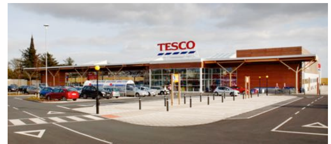
TESCO Eco Store – The first Passivhaus supermarket in the world was created in 2008 in Tramore, Ireland. It has solar photovoltaic panels and a ground source heat pump that provides water heating from waste heat taken from the cooling cabinets. ©Joseph Doyle Architects
