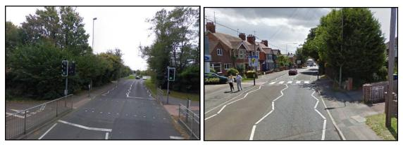
Bucknell Road has footways along both sides of the carriageway, varying in width between 1.2 and 2.0 metres, which is substandard in places. The footways do generally benefit from a good horizontal alignment, street lighting, appropriate crossing infrastructure and a well maintained surface condition.
