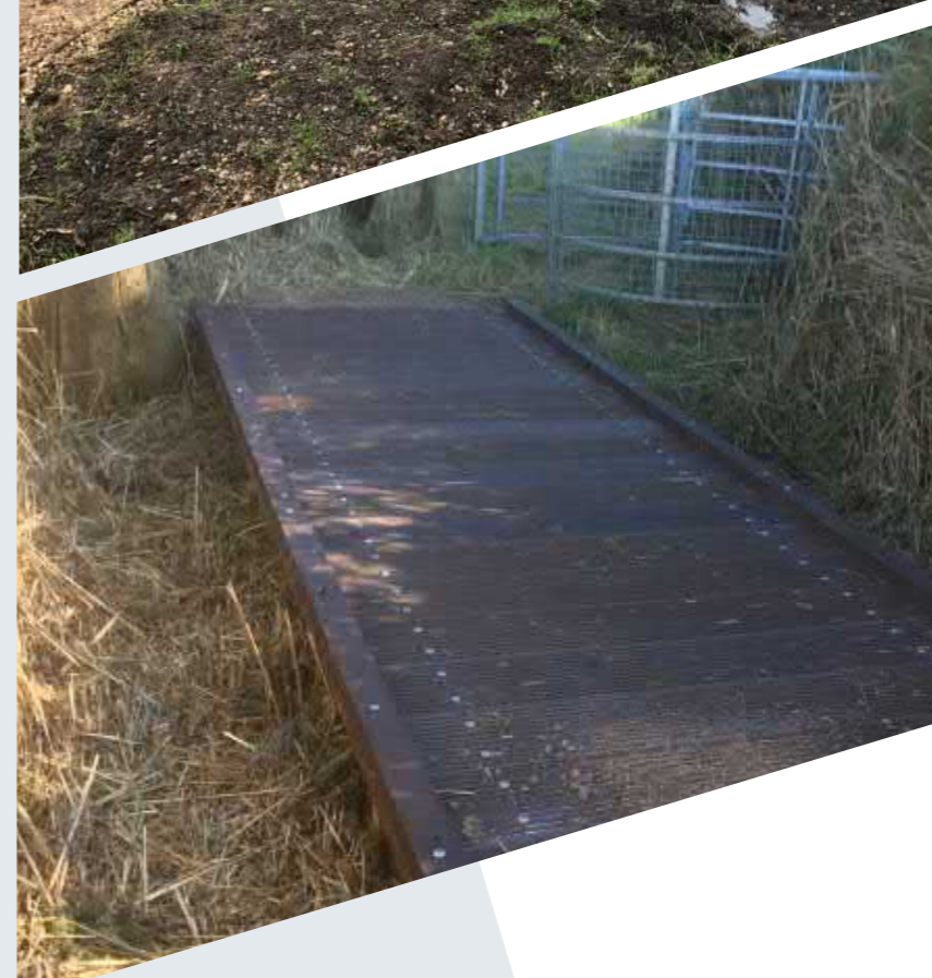
5mm near diamond hard gritted surface with a recycled bottle core on planks.
