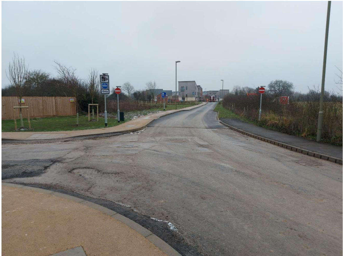
Figure 4-8: Existing Bus Gate within the Exemplar Scheme
