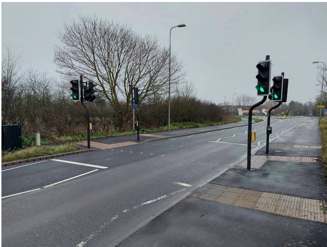
Figure 4-2: Existing Toucan crossing on the B4100 Banbury Road
