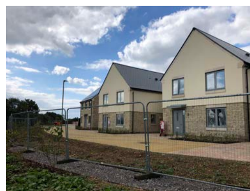
New homes under construction in phases 3 and 4 for the Exemplar Site
