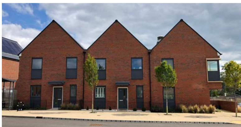
Terraces at the Exemplar Site
