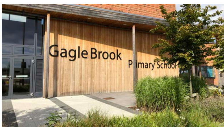
Gagle Brook Primary School is close to the Site
