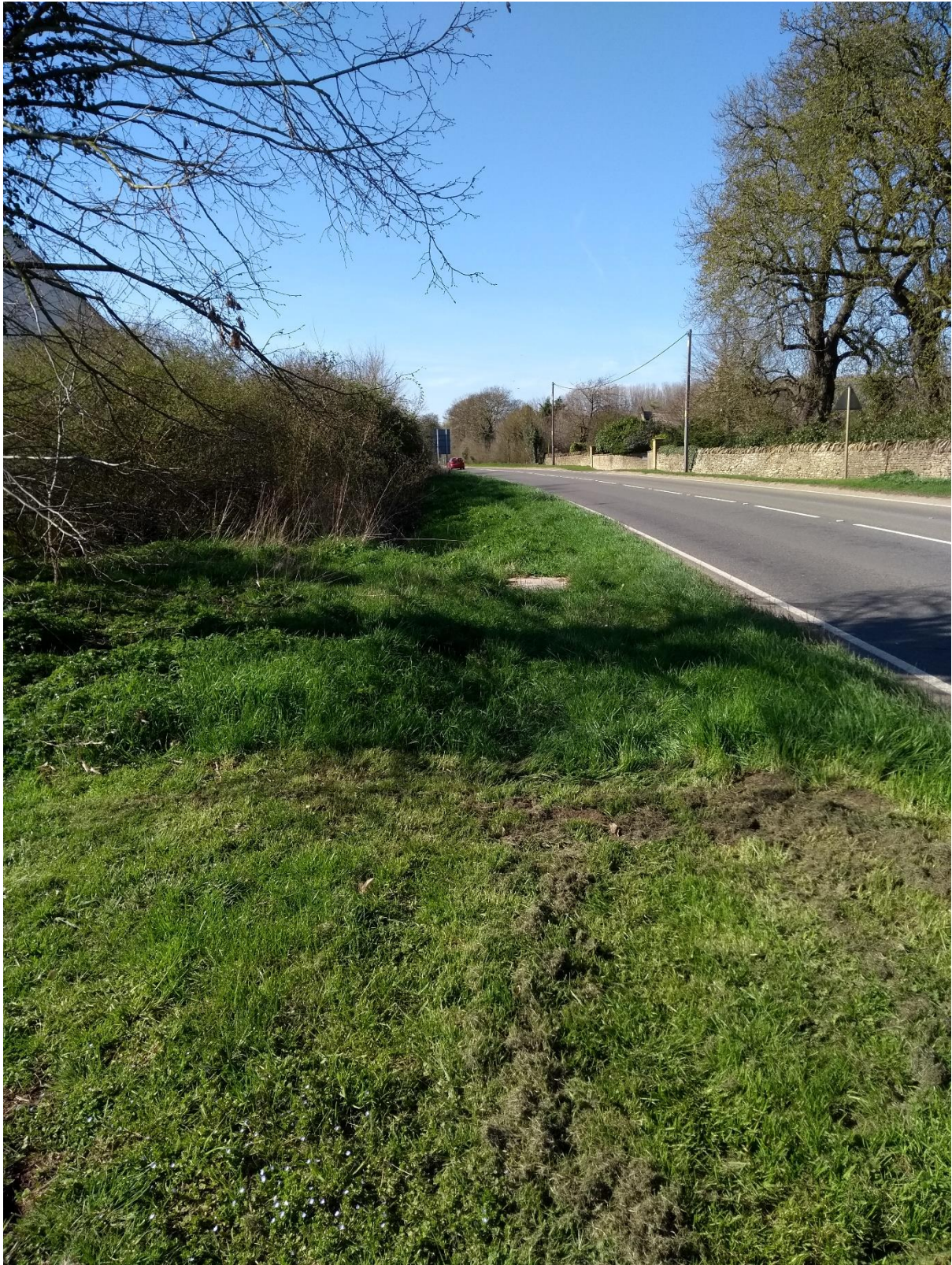
Figure 5: Figure 4: View looking West along the B4100, standing 2.4 metres back from the road edge at the location of the proposed Access E. The drain discussed in this report, located within 2.20 metres from the road edge, can be seen via the light coloured access hatch in mid-picture. The ditch is overgrown currently with weeds; the hedge is actually further to the left: this all simply needs trimming back to restore the visibility splay 'in perpetuity' for Home Farm.
