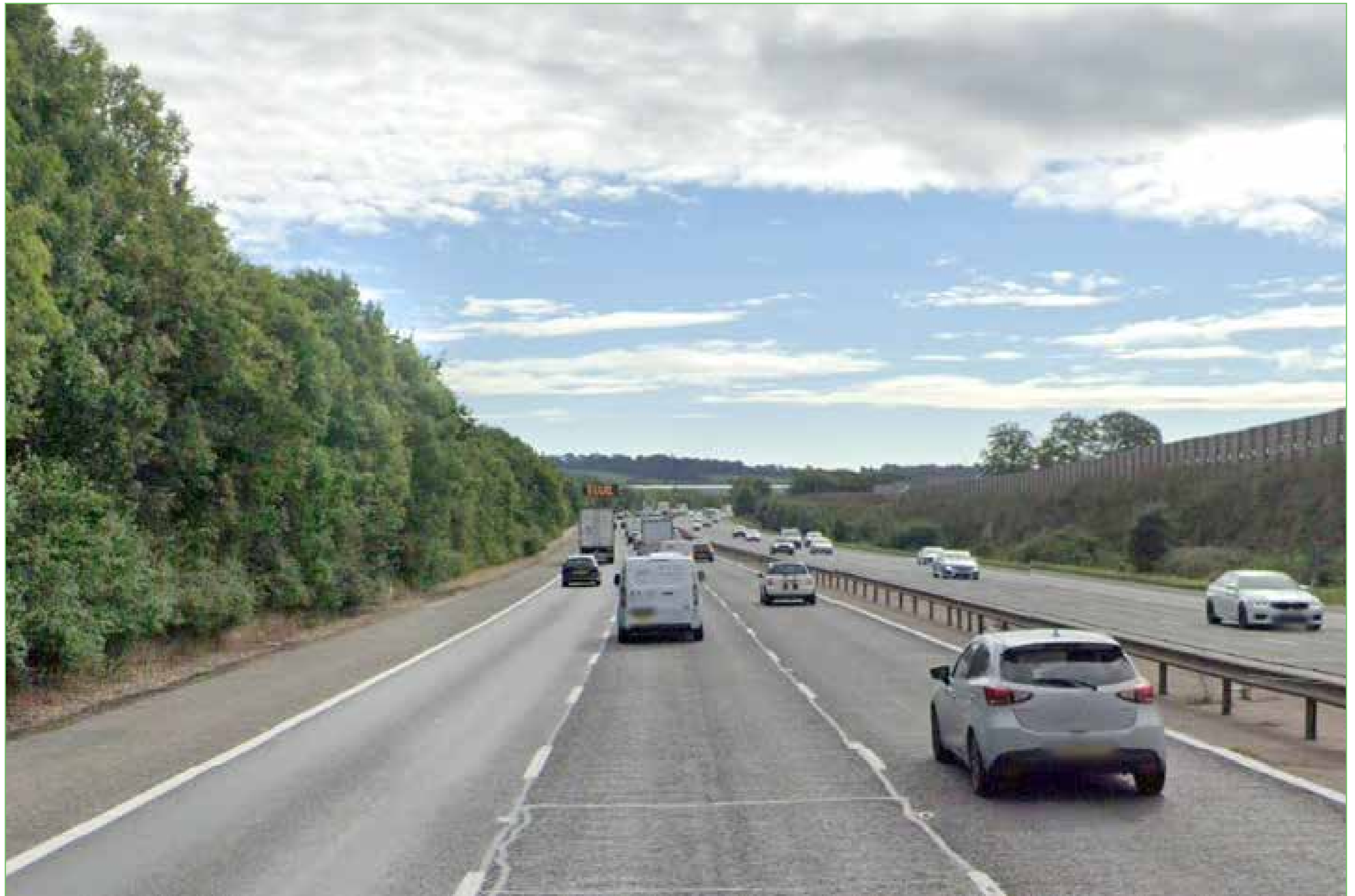
Appendix 5.1, Figure 5.34 Viewpoint Photograph 16 - Google Streetview capture 21340 Land East of Junction 11, M40, Banbury
