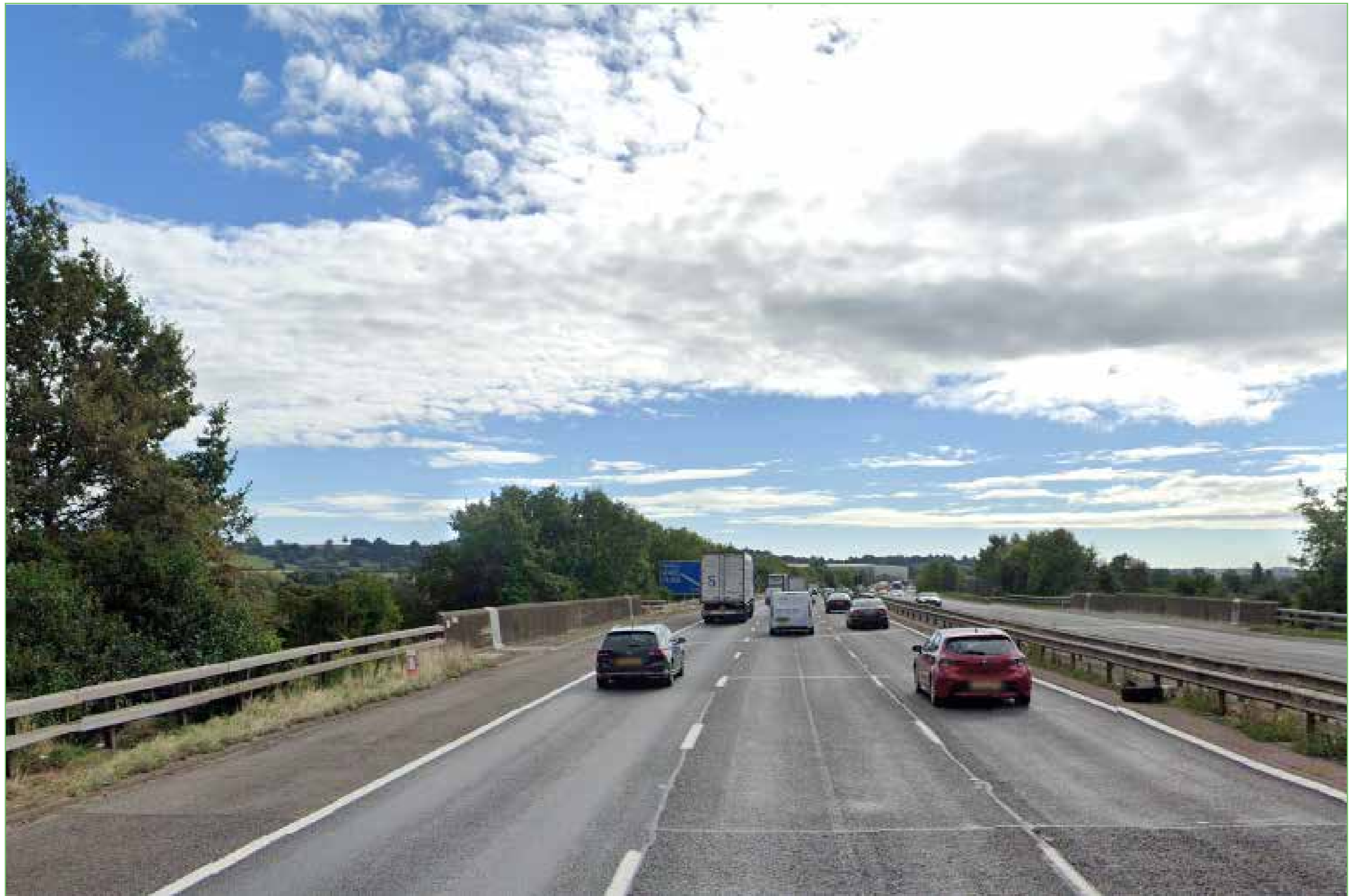
Appendix 5.1, Figure 5.33 Viewpoint Photograph 15 - Google Streetview capture 21340 Land East of Junction 11, M40, Banbury
