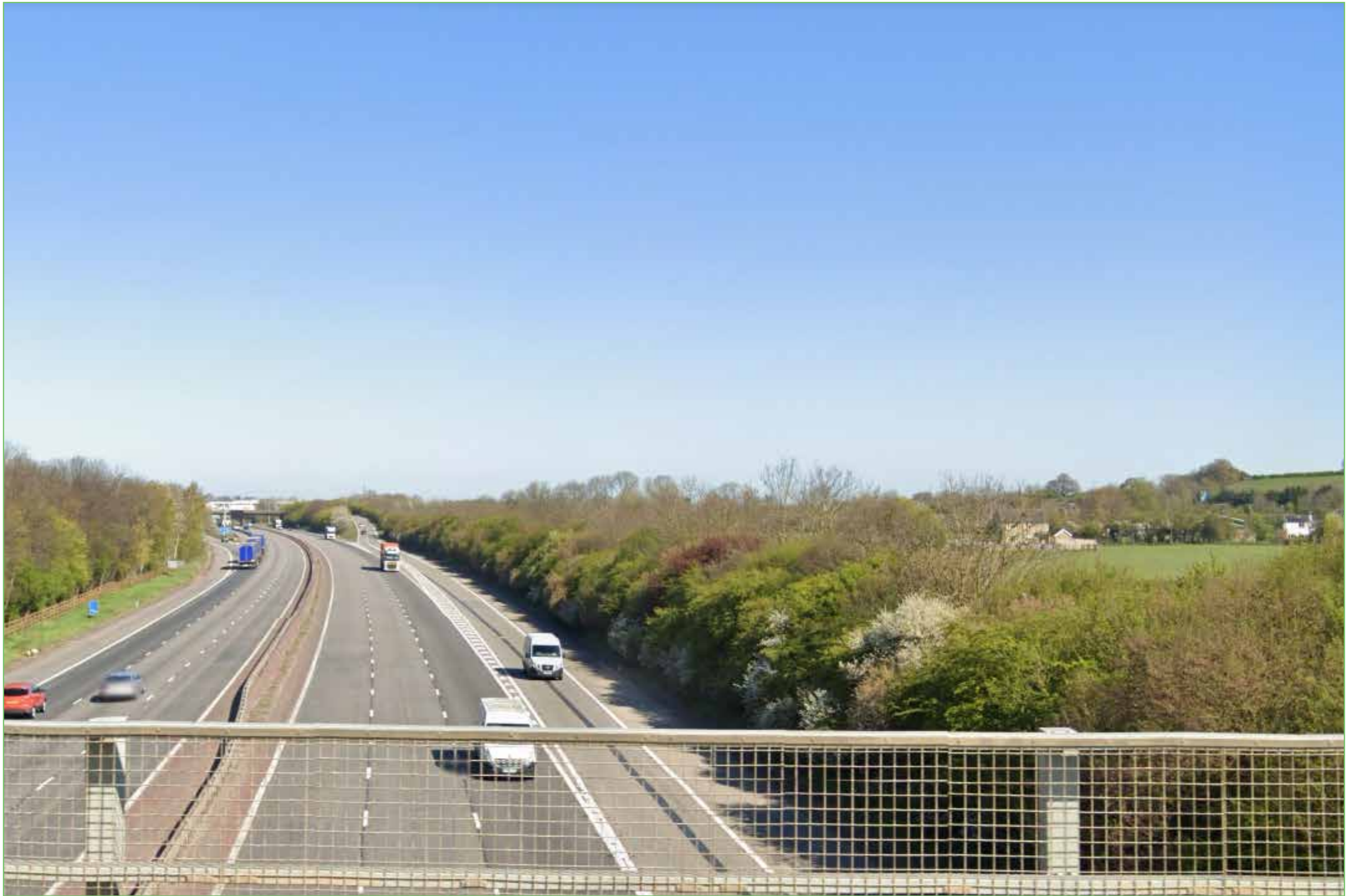
Appendix 5.1, Figure 5.31 Viewpoint Photograph 13 - Google Streetview capture 21340 Land East of Junction 11, M40, Banbury
