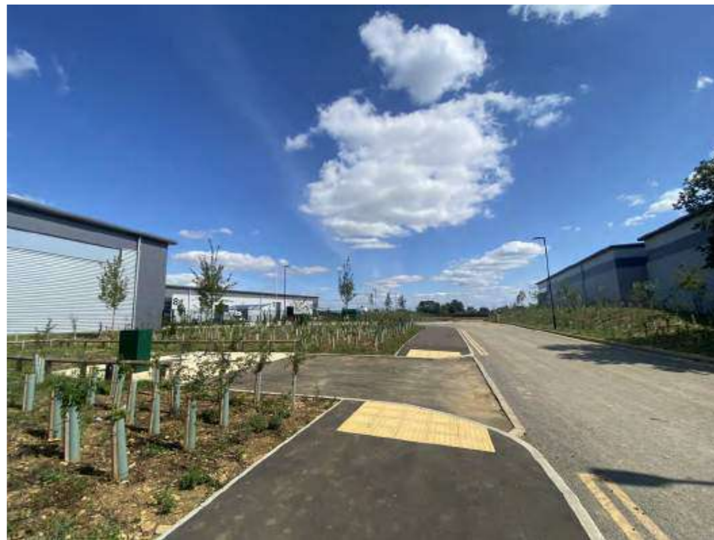
Fig. 06 Looking South East on temporary initial road
