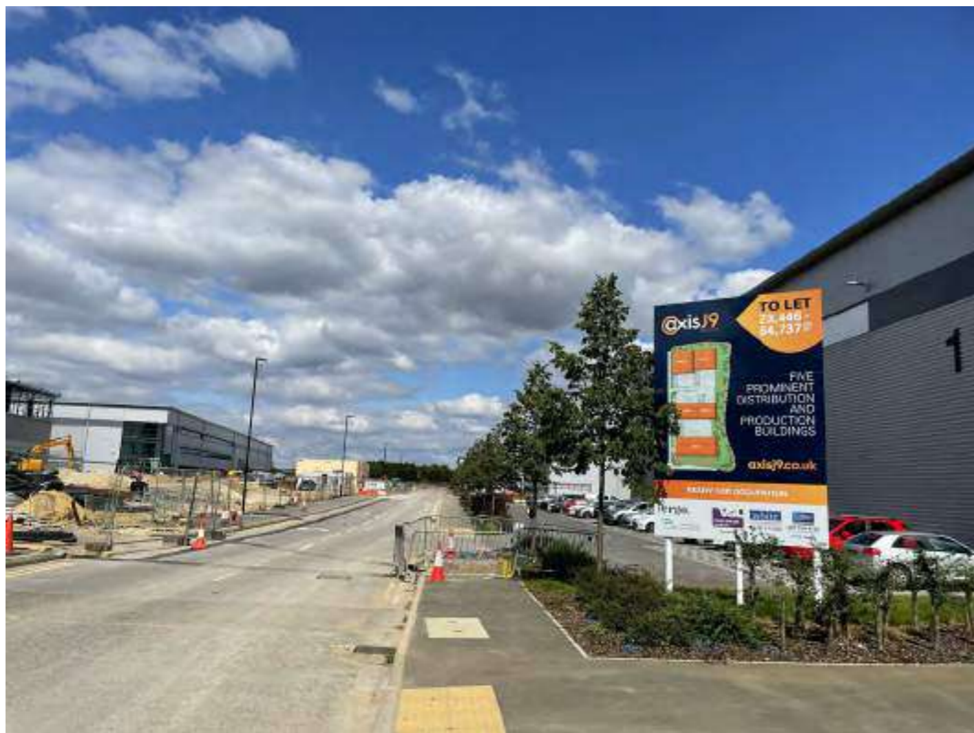
Fig. 05 Looking North East on initial access road
