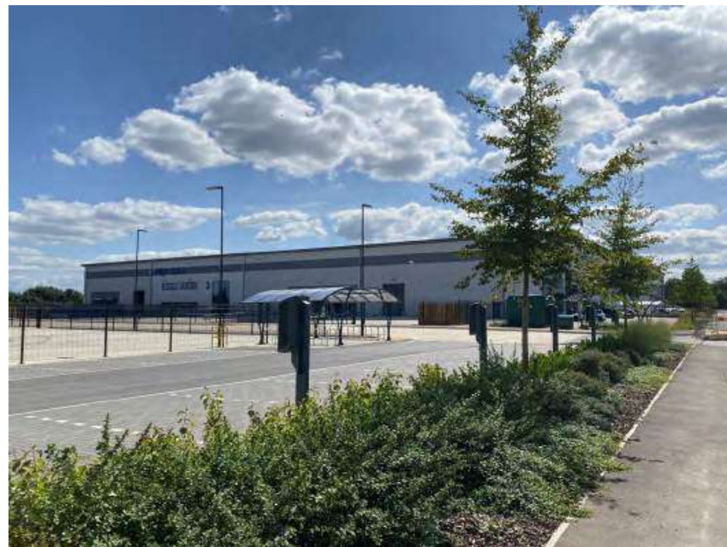
Fig. 08 Units 2 & 3 viewed from Empire Road (Access Road)
