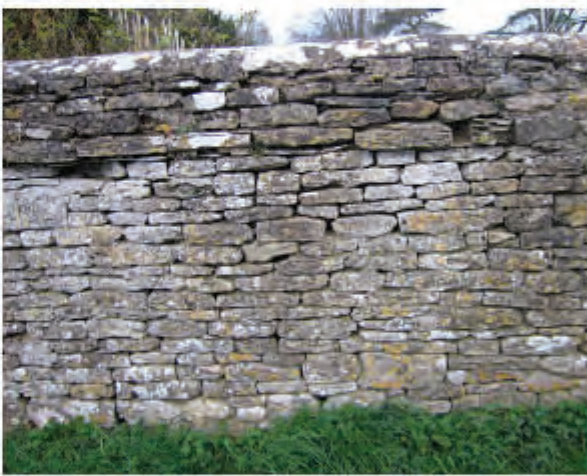
Heaped mortar forms coping
