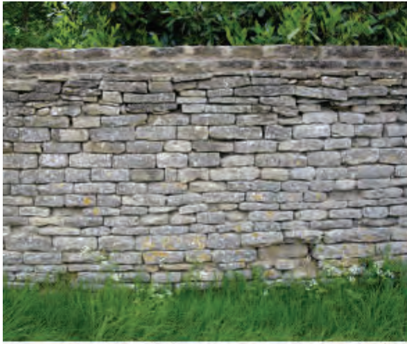
Mortared stone course forms coping
