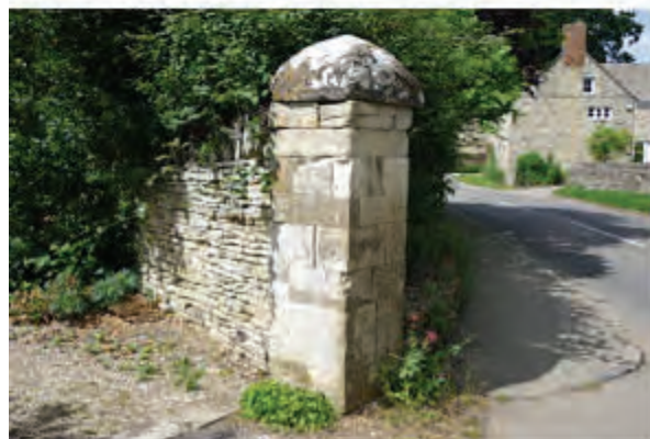
Impressive stone entrance pier outside Gossway
