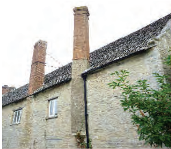
External chimney at the Manor House
