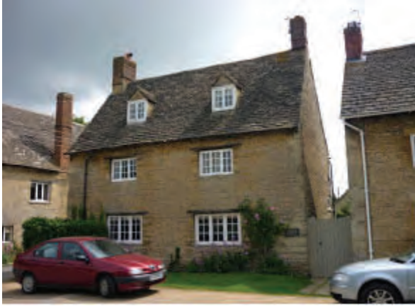
The Green Cottage/ Church Cottage
