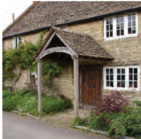
Porch on the Old Bakehouse.
