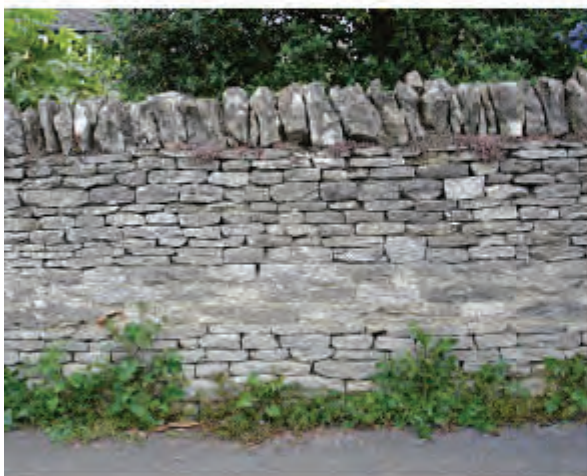
Stone laid on edge forms coping
