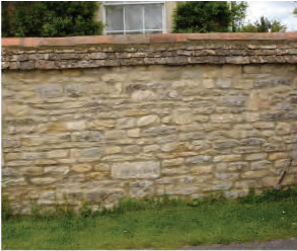
Tiles and stone slates form coping
