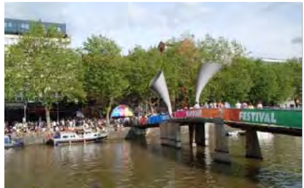
Bridge in Bristol Harbourside
