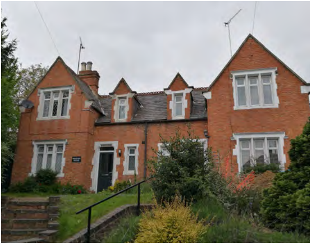
Union Master's House, Warwick Road
