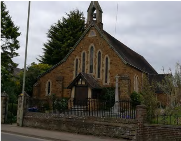
St. Paul's Church Warwick Road
