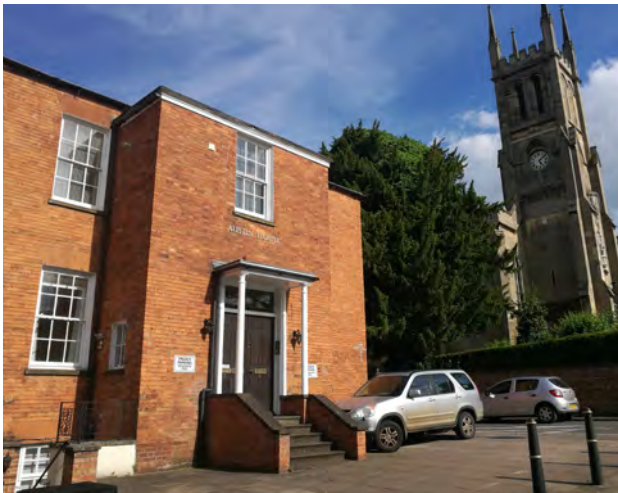
Austin House South Bar Street
