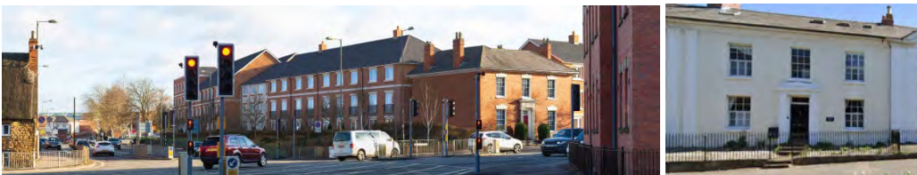
Railings Oxford Road
