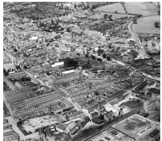
View NW across Newlands 1929 ( Banbury Town Hall, the Britannia Works and Hunt Edmunds Brewery ( now both demolished) centre picture, canal in the foreground)
