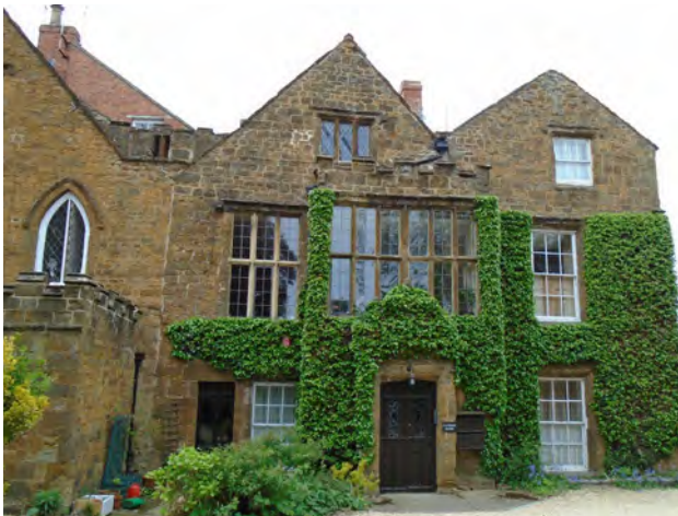
Calthorpe Manor (17th Century wing)
