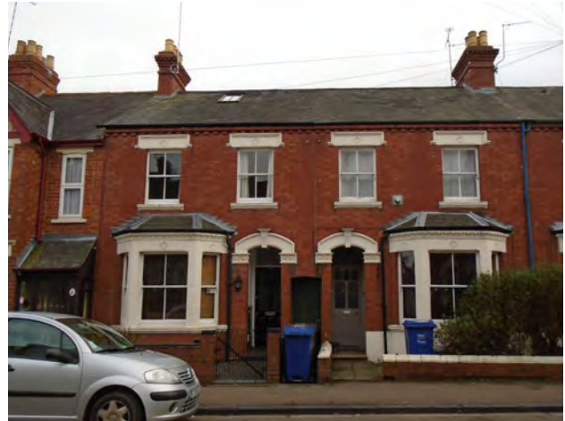
Queens Road 19th Century terrace housing
