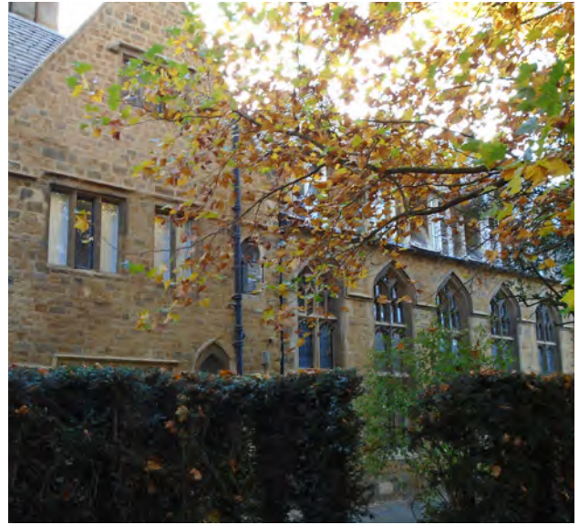
Church room to the rear of 24 Horse Fair
