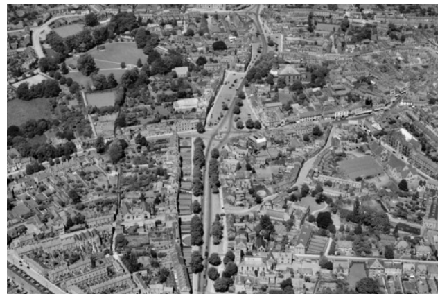
View North 1947 ( West Bar Street area bottom left, Court House centre top of picture)
