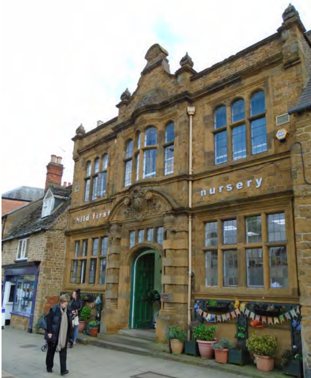
Former offices of the Poor Law Guardians (now nursery)
